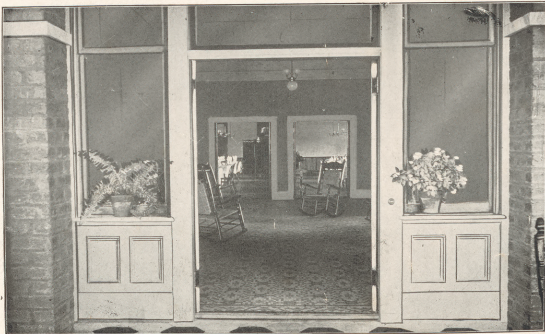
Main Entrance Lanier Hall.
