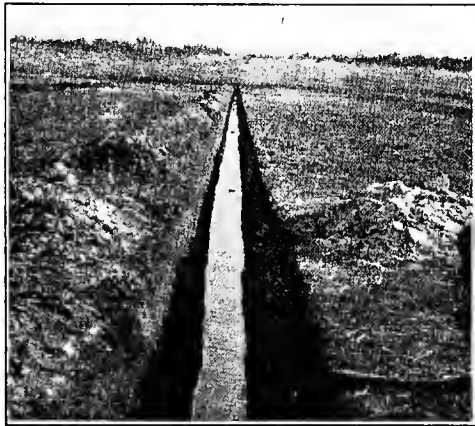
FIG. 19. — An open drainage ditch in muck soil in New Jersey.
