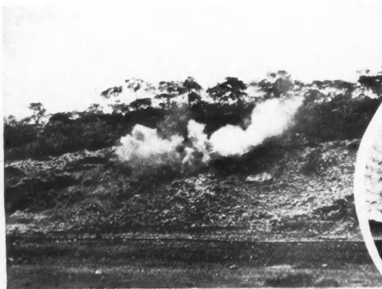
Stripping at Bwana M'Kubwa copper mine, Northern Rhodesia
