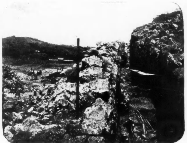
Stoped-out high-grade vein, Bwana M'Kubwa mine A large tonnage of low-grade ore adjoins this
