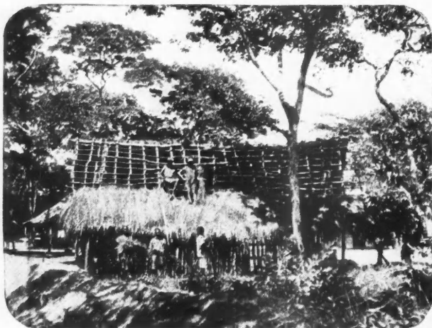
Building construction at N'Kana mine, Northern Rhodesia
