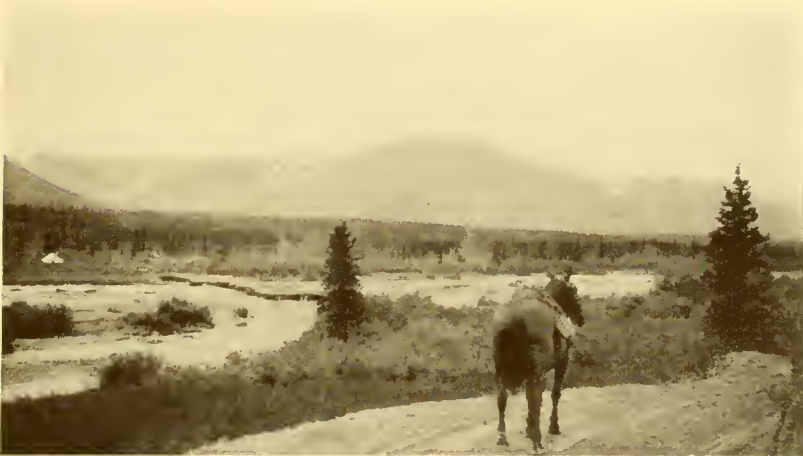
FIG. 63.—Middle fork of Chulitna, a little south of Broad Pass. Corduroy bridge of the Alaskan Engineering Commission.
