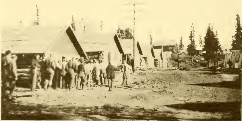
FIG. 62.—Hurricane, a construction camp on the government railroad 285 miles north from Seward, Alaska.
