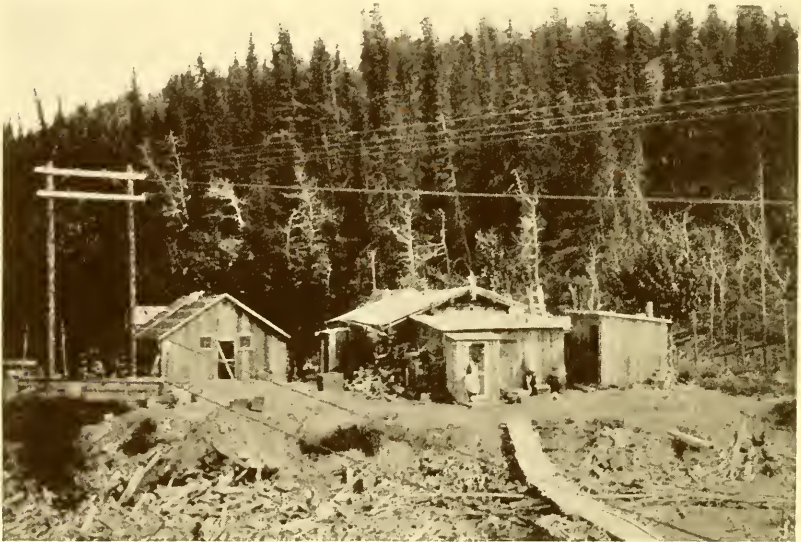
FIG. 67.—Construction camp at Nenana Bridge, north of Healy, Alaska.
