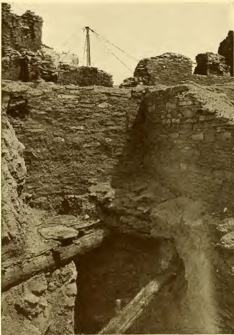
FIG. 136.—Dwellings in Pueblo Bonito were sometimes razed to permit of the construction of ceremonial chambers. The former ceiling beams shown in this illustration are here used both as braces for the curved wall of a kiva and as supports for a second-story room which was subsequently abandoned as its enclosing walls were still further altered. (Photograph by Neil M. Judd. Courtesy of the National Geographic Society.)
