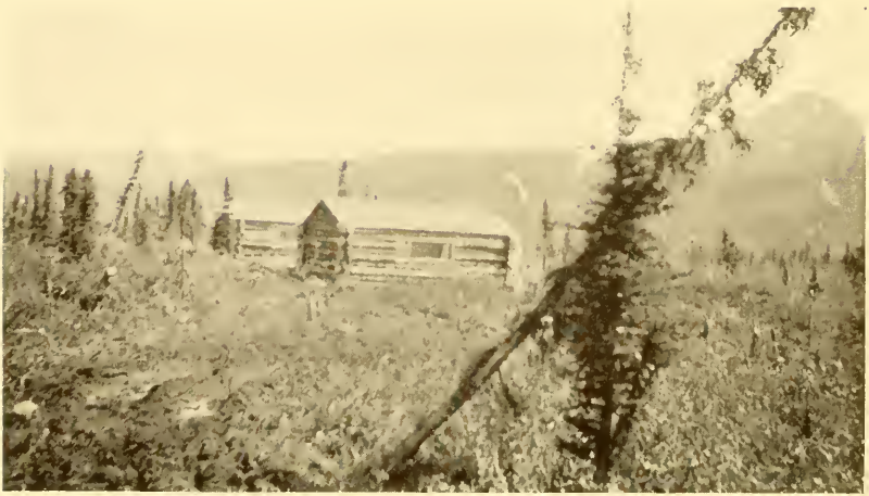
FIG. 64.—Contractors' cabins on the line of the government railroad near Broad Pass, Alaska.
