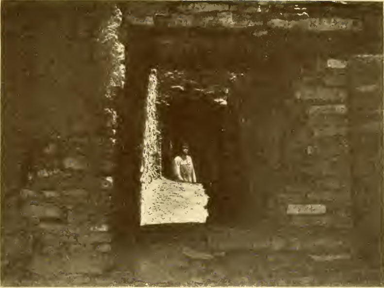
FIG. 129.—A narrow, elevated passage-way constructed through one Pueblo Bonito room to connect the two adjoining chambers. The lintel poles of the nearer doorway are supported, on the right, by a hewn plank which rests upon an upright pine log partially imbedded in the wall. (Photograph by Neil M. Judd. Courtesy of the National Geographic Society.)
