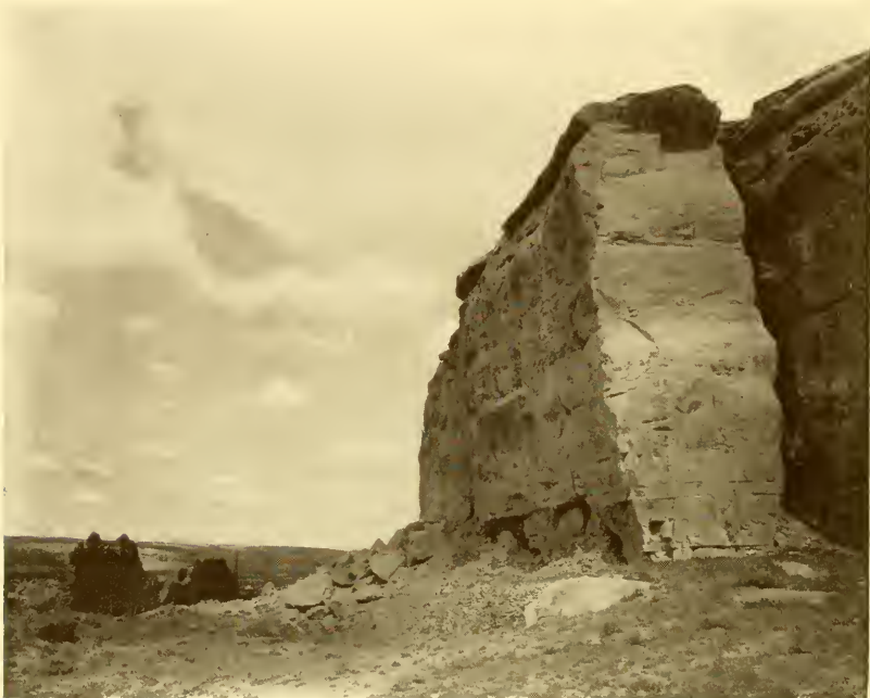
FIG. 121.—A naïve example of Bonitian engineering. In an obvious attempt to hold up a huge section of cliff which threatened to topple upon their village, the ancients placed pine props under the weathered section and covered these with a great terraced mass of masonry. The north wall of Pueblo Bonito stands at the left. (Photograph by Charles Martin. Courtesy of the National Geographic Society.)
