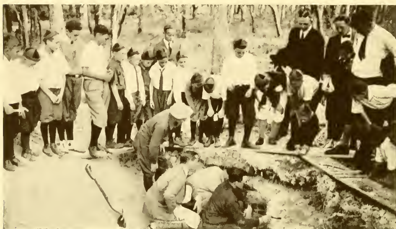
FIG. 85.—Boy Scouts watching progress of excavations, Weeden Mound, Florida.
