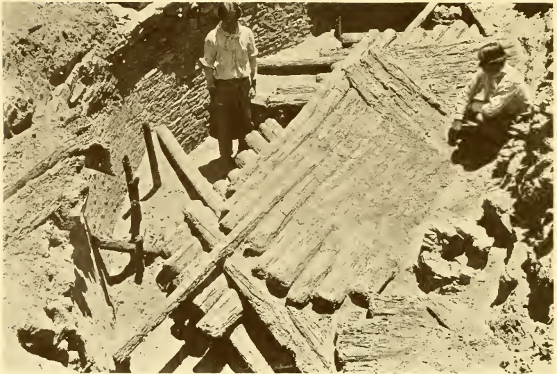
FIG. 60.—The roof of a Pueblo Bonito council chamber was a very complicated affair. Beginning on eight or ten low masonry supports, pairs of logs lay close to the kiva wall; above these were other poles laid in threes, fours, etc., until a neat vault, flat on top, covered the room. (Photograph by O. C. Havens. Courtesy of the National Geographic Society.)
