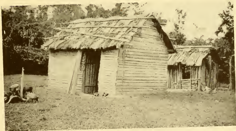
FIG. 44.—A typical house near Jovero. The roof is formed of the sheathing leaf-bases of the royal palm ( Roystonea ).
