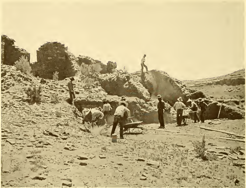
FIG. 72.—This view of work in progress on the west side of Pueblo del Arroyo illustrates the extent to which fallen masonry and blown sand will accumulate. (Photograph by O. C. Havens, Courtesy of the National Geographic Society.)
