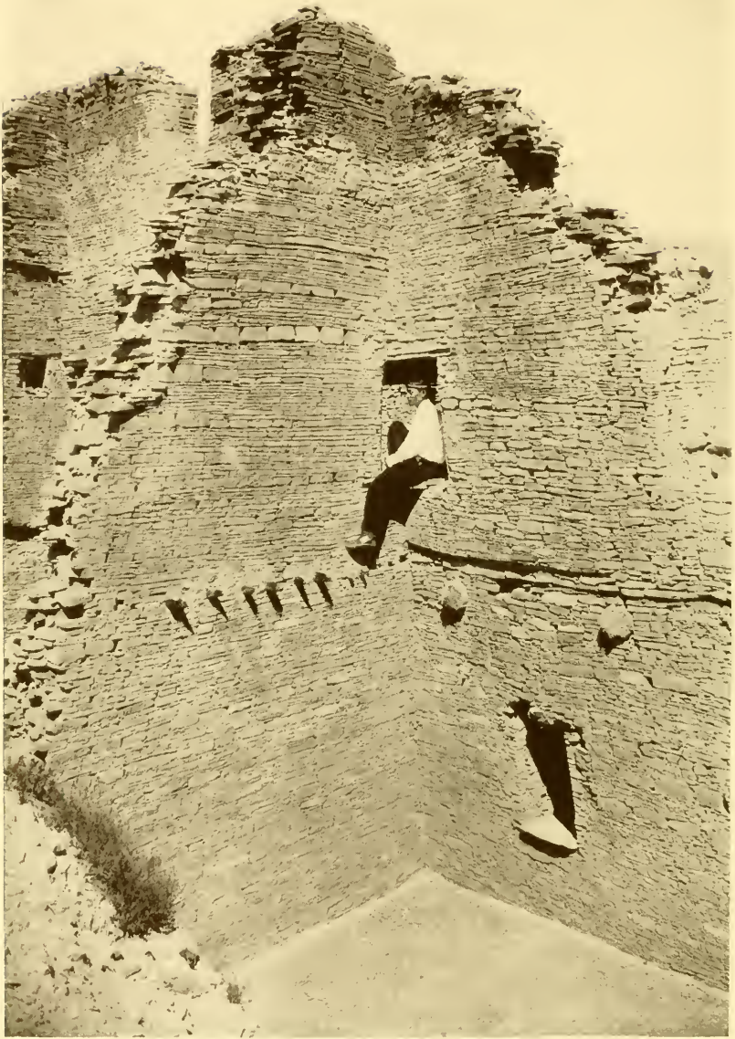
FIG. 117.—Repaired walls of the third type of masonry, showing occasional bands of thicker blocks inserted for strength and decorative effect. Corner doorways are not uncommon in Pueblo Bonito; they provided a direct means of communication between neighboring dwellings occupied by members of the same family or clan. (Photograph by Neil M. Judd. Courtesy of the National Geographic Society.)
