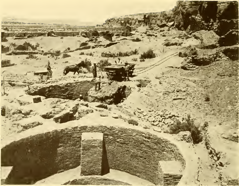
FIG. 131.—Excavating one of Pueblo Bonito's numerous kivas. Mule-drawn dump cars were used in connection with a portable steel track which could be shifted as the explorations progressed. Owing to the depth of some rooms it was necessary to pass the debris upward from one man to another before it reached the track level. (Photograph by Neil M. Judd. Courtesy of the National Geographic Society.)
