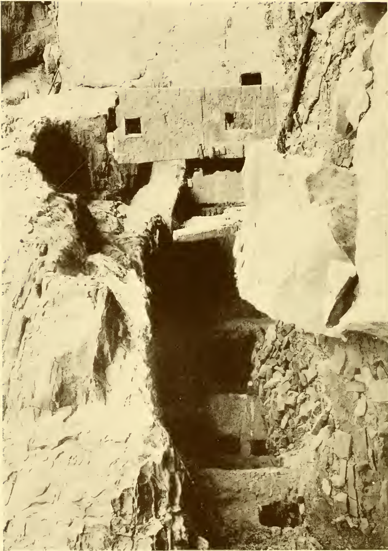
FIG. 76.—Oak-tree House, before repair. (Photograph by Geo. L. Beam. Courtesy Denver and Rio Grande Railroad.)
