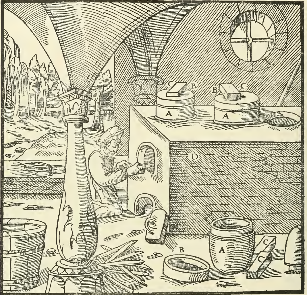
A—POTS. B—LIDS. C—STONES. D—FURNACE.
