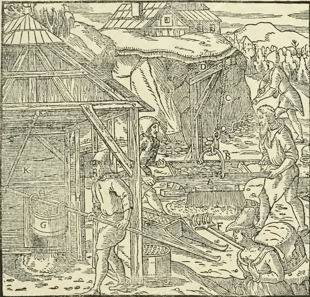
A—BOX. B—BALE. C—ROPE. D—BEAM. E—HANDLES. F—FIVE-TOOTHED RAKE. G—SIEVE. H—ITS HANDLES. I—POLE. K—ROPE. L—TIMBER.
