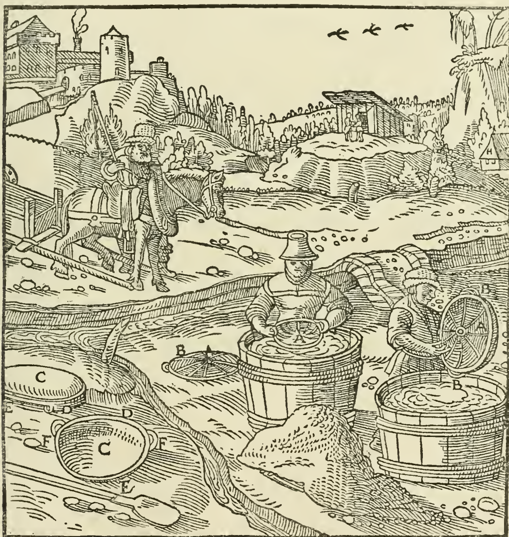
A—BASKET. B—ITS HANDLES. C—DISH. D—ITS BACK PART. E—ITS FRONT PART. F—HANDLES OF SAME.
