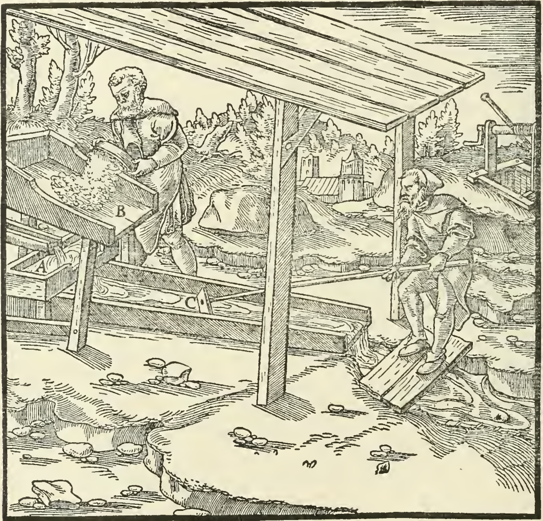
A—TROUGH. B—PLATFORM. C—WOODEN SCRUBBER.
