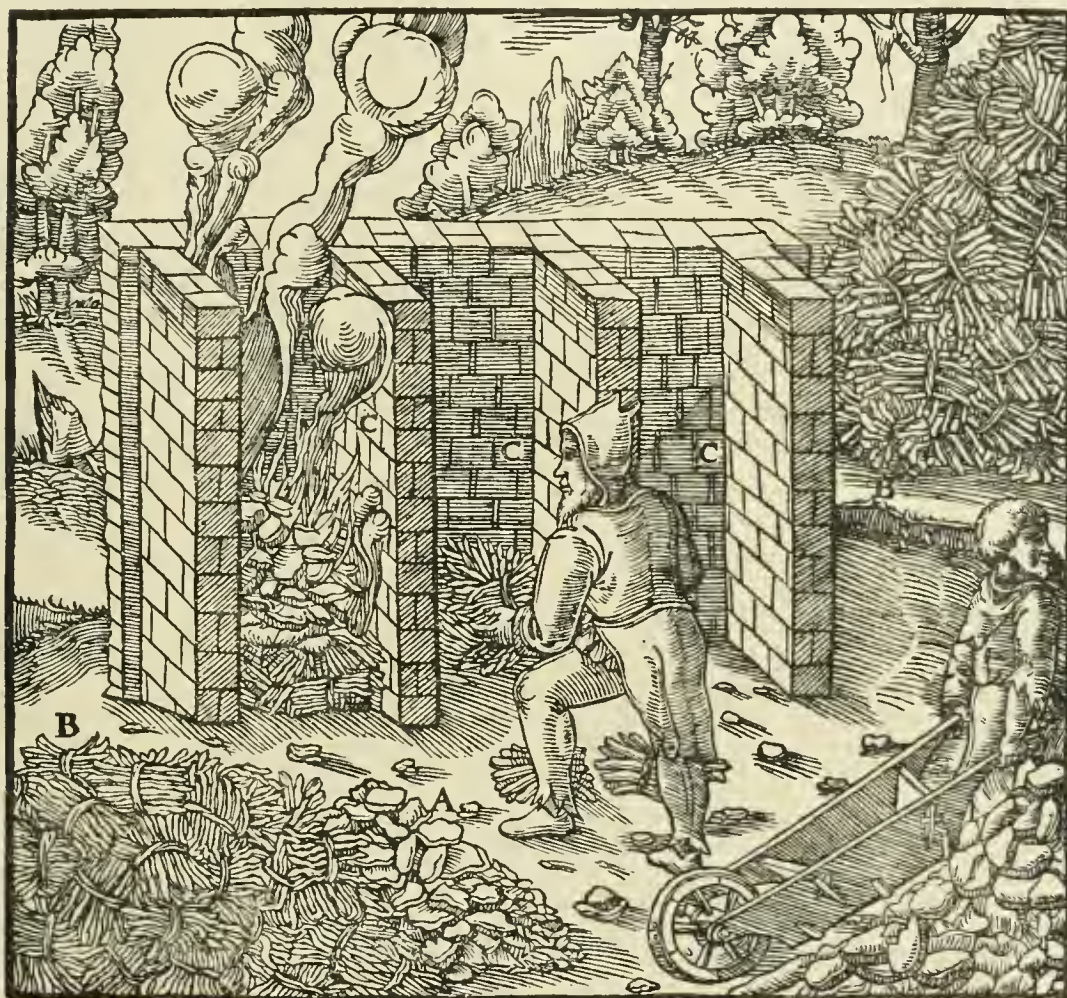
A—CAKES. B—BUNDLES OF FAGGOTS. C—FURNACES.
