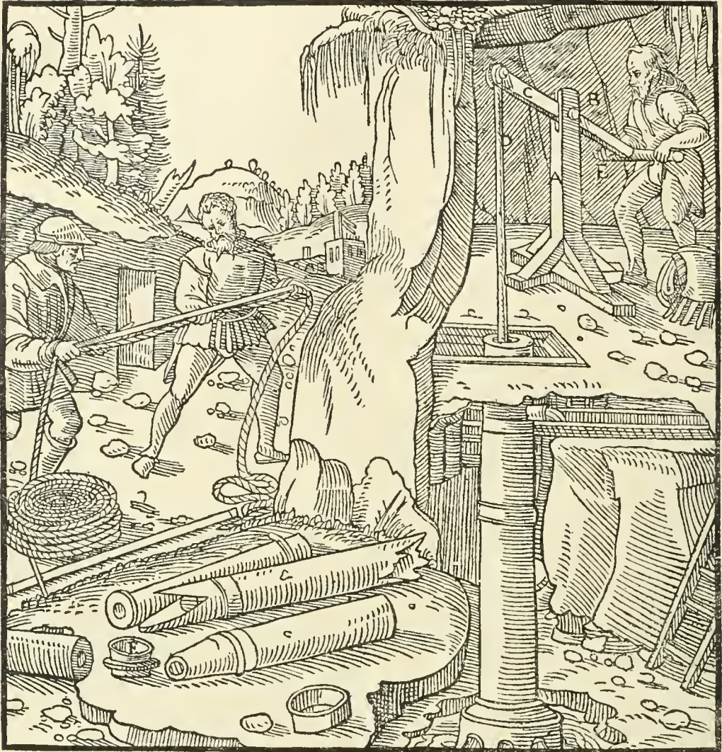
A—ERECT TIMBER. B—AXLE. C—SWEEP WHICH TURNS ABOUT THE AXLE. D—PISTON ROD. E—CROSS-BAR. F—RING WITH WHICH TWO PIPES ARE GENERALLY JOINED.
