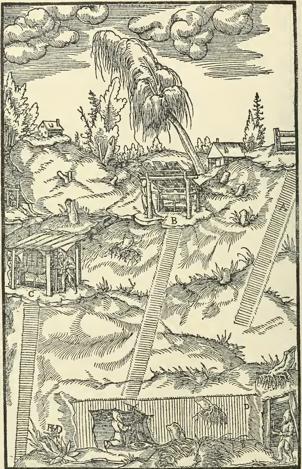
THREE INCLINED SHAFTS, OF WHICH A DOES NOT YET REACH THE TUNNEL; B REACHES THE TUNNEL; TO THE THIRD, C, THE TUNNEL HAS NOT YET BEEN DRIVEN. D—TUNNEL.
