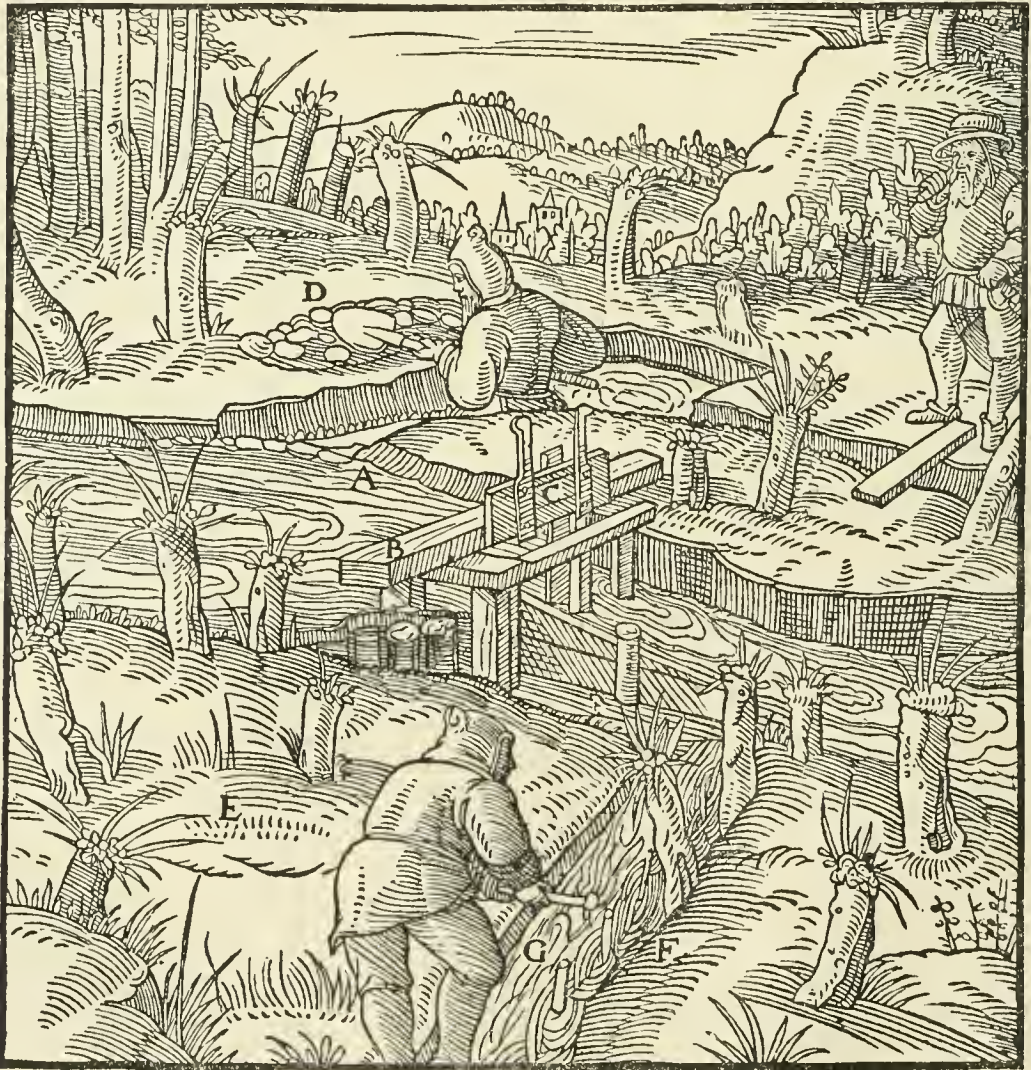
A—RIVER. B—WEIR. C—GATE. D—AREA. E—MEADOW. F—FENCE. G—DITCH.
