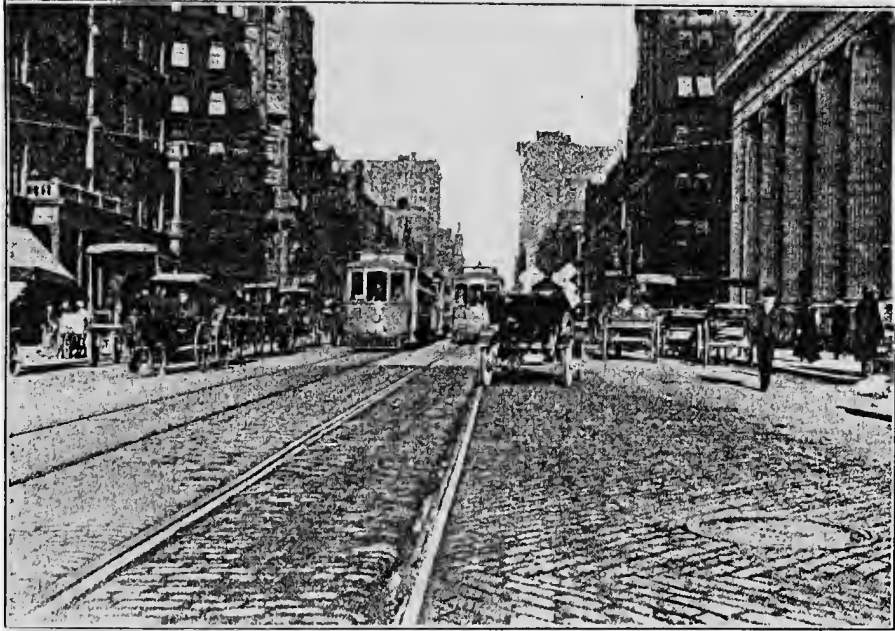
MAIN STREET, LOOKING EAST.
