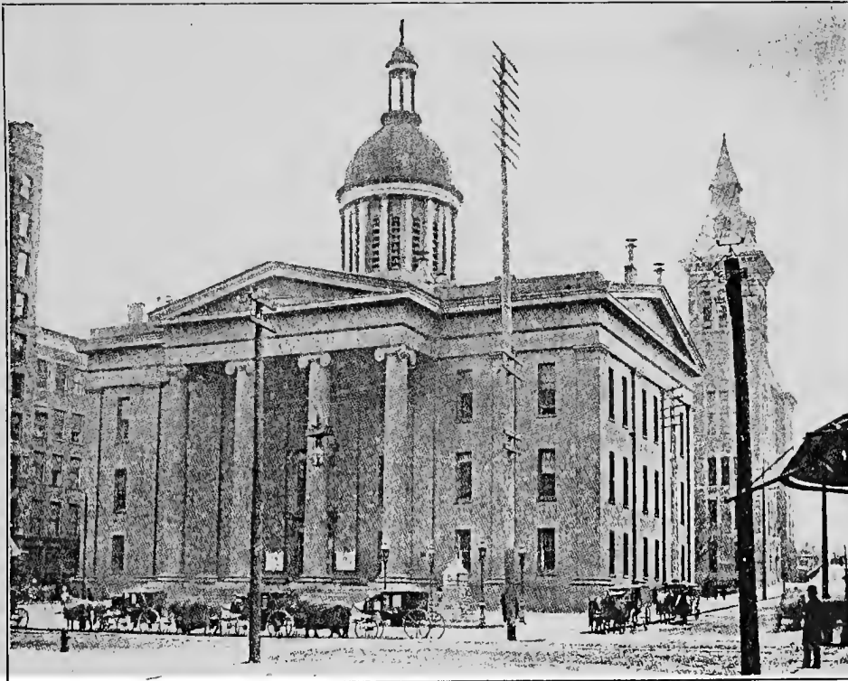
SECOND MONROE COUNTY COURT HOUSE.
