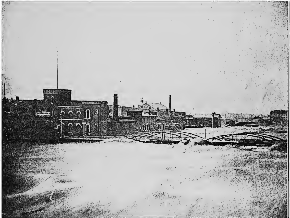
THE FLOOD OF 1865. ANDREWS STREET BRIDGE.
