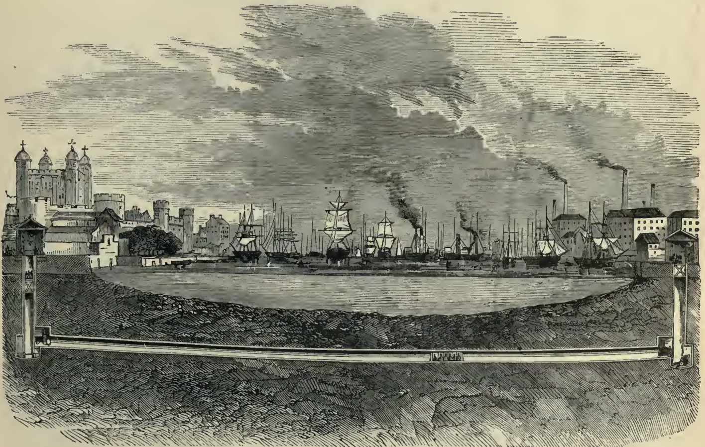
THE NEW TOWER SUBWAY, UNDER THE RIVER THAMES.
