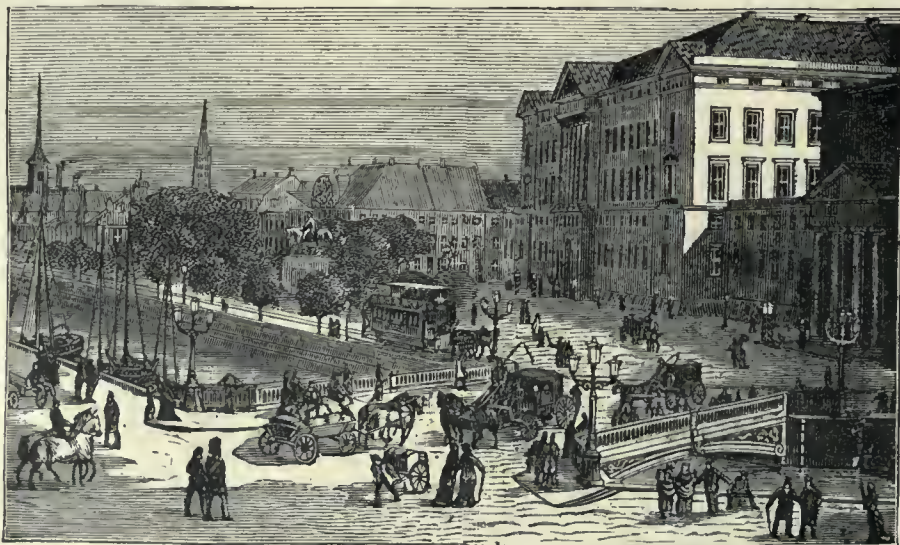
THE SLOTSHOLM SIDE OF COPENHAGEN—THE NEW CANAL BRIDGE.
