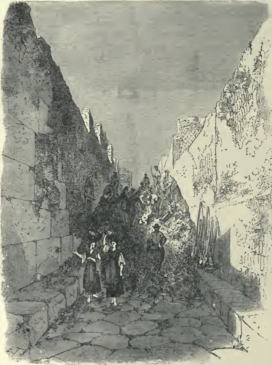
EXCAVATION IN A STREET AT POMPEII.
