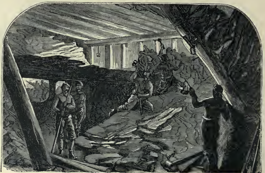
RAILWAY TUNNEL OF THE ALPS—SECOND AND THIRD GALLERIES OF THE TUNNEL EXCAVATION.
