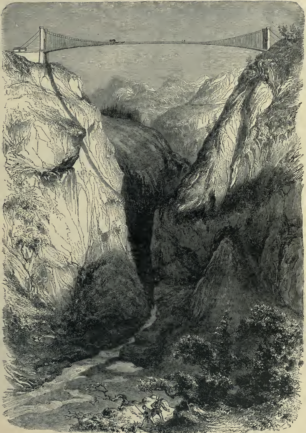
CAILLE BRIDGE, IN SAVOY.
