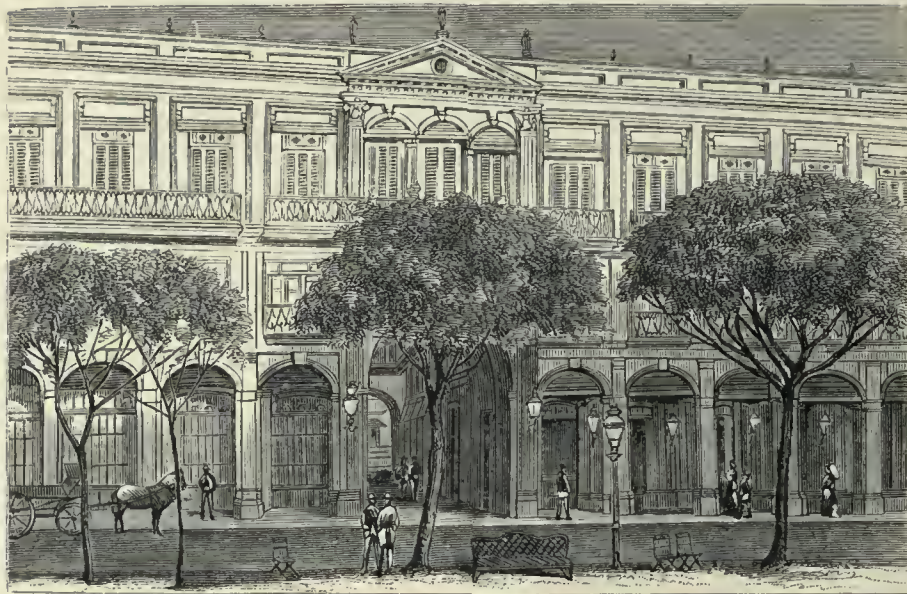
EXTERIOR OF THE HOTEL PASAGE, HAVANA.
