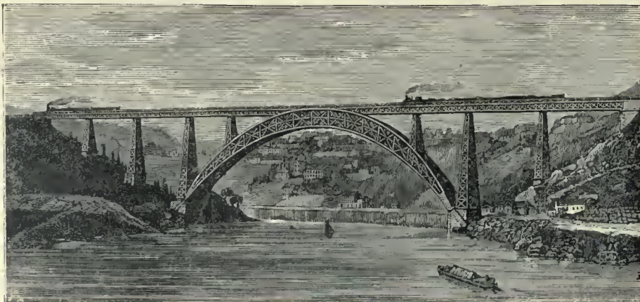
BRIDGE AT PORTO.
