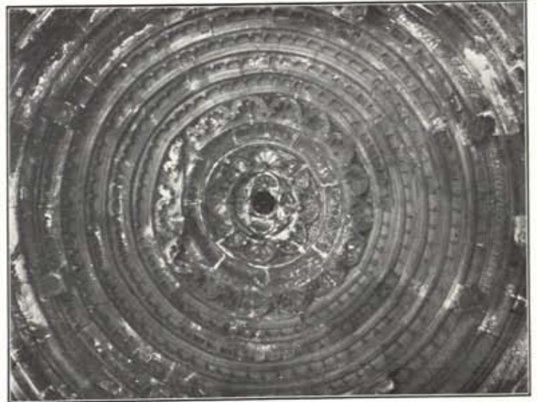
(b) VIEW OF DOMED HINDU CEILING OF COLONNADE IMMEDIATELY BEHIND THE EAST ENTRANCE GATE OF QUTBU-D-DIN'S MOSQUE.
