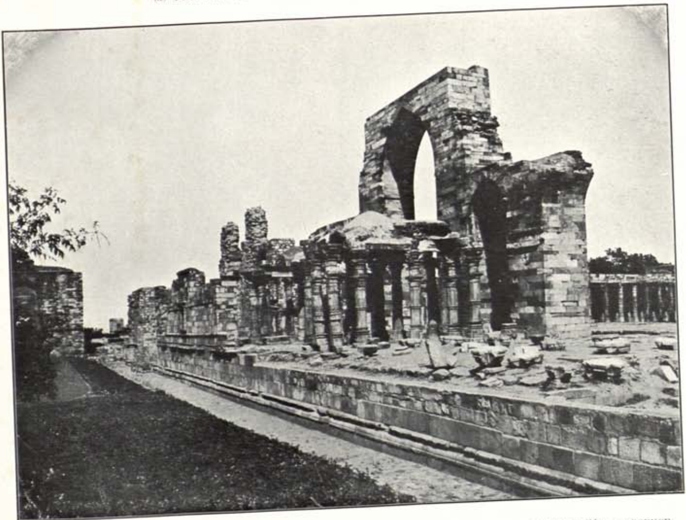
(b) VIEW OF QUTBU-D-DIN'S ORIGINAL MOSQUE FROM S.W., SHOWING RUINS OF PRAYER CHAMBER (NOTE ABSENCE OF ANY MIHRAB PROJECTION IN THE CENTRE OF PLINTH, AND COMPARE SIMILAR FEATURE IN ALTAMISH'S EXTENSION, WHERE MIHRAB PROJECTION DOES EXIST; (PLATE No. 5 b)).
