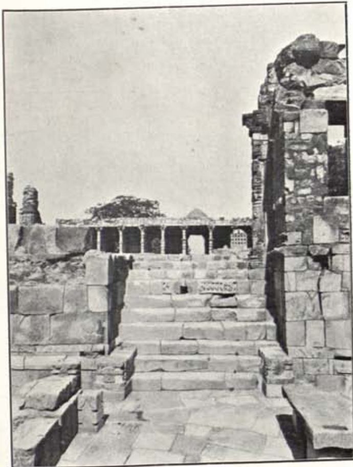
(c) SOUTH GATE OF QUTBU-D-DIN'S ORIGINAL MOSQUE, SHOWING "RETURN" OF PLINTH-MOULDING ON WEST JAMB ONLY. ITS OMISSION FROM THE CORRESPONDING EAST JAMB IS A FACTOR SUPPORTING THE ASSUMPTION THAT THE CHABUTRA WEST OF THIS GATE IS OF THE ORIGINAL TEMPLE.
