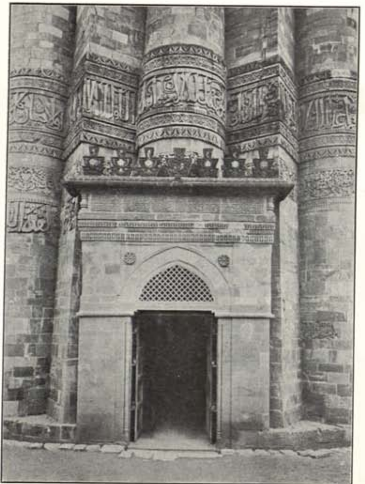
(c) MINAR. ENTRANCE DOORWAY (REPAIRED BY MAJOR SMITH, R.E. IN 1828). ALL THE WORK ABOVE THE ARCHITRAVE IS THE ORIGINAL REPLACED IN POSITION.
