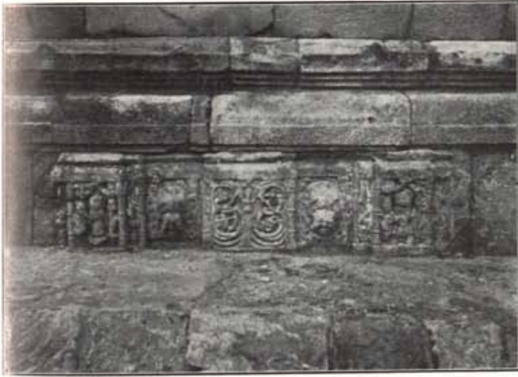
(a) DETAIL OF HINDU SCULPTURED LINTEL BUILT UPSIDE-DOWN IN THE PLINTH OF QUTBU-D-DIN'S MOSQUE EAST OF THE NORTH GATEWAY; THUS PROVING THE MUHAMMADAN ORIGIN OF THIS PORTION OF THE CHABUTRA.
