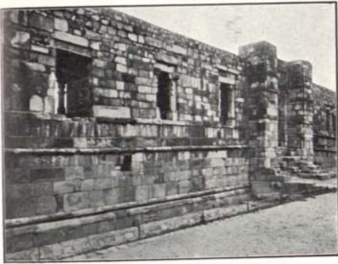
(a) QUTBU-D-DIN'S ORIGINAL MOSQUE. EASTERN HALF OF NORTH FACADE, SHOWING HINDU CARVED STONES BUILT INTO PLINTH, AND ALSO SCULPTURED LINTEL PORTRAYING "BIRTH OF KRISHNA" OVER UPPER WINDOW.
