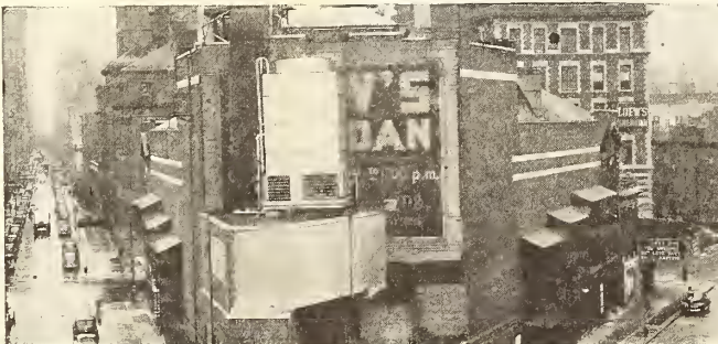
Cooling tower atop Loew's Sheridan Theatre, New York City.
