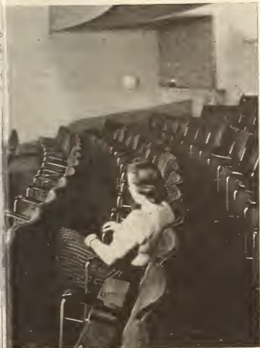
View of one of the newer theatres in Finland (Turku Abo; Eric Bryggman, architect) in which wide row spacing is employed to provide easy access and safety without limiting the number of seats per row, as suggested in the preferred plans presented in this issue.
