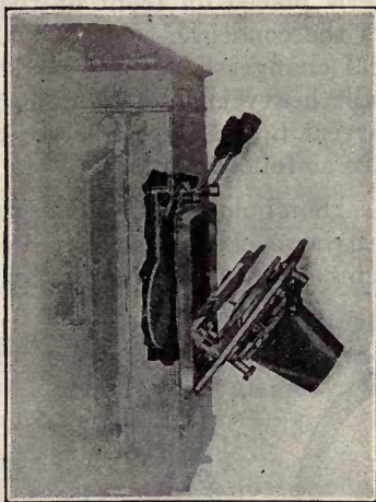
Close-Up of Condenser Mount and Holder, and Adjustment for Inside Dowser
