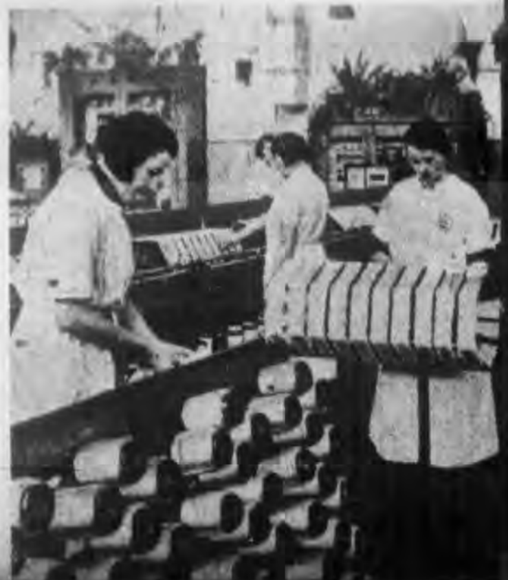
○起捲管絲捲用，後之乾晒 When it emerges from the drying chamber, the artificial silk is spooled on bobbins.
