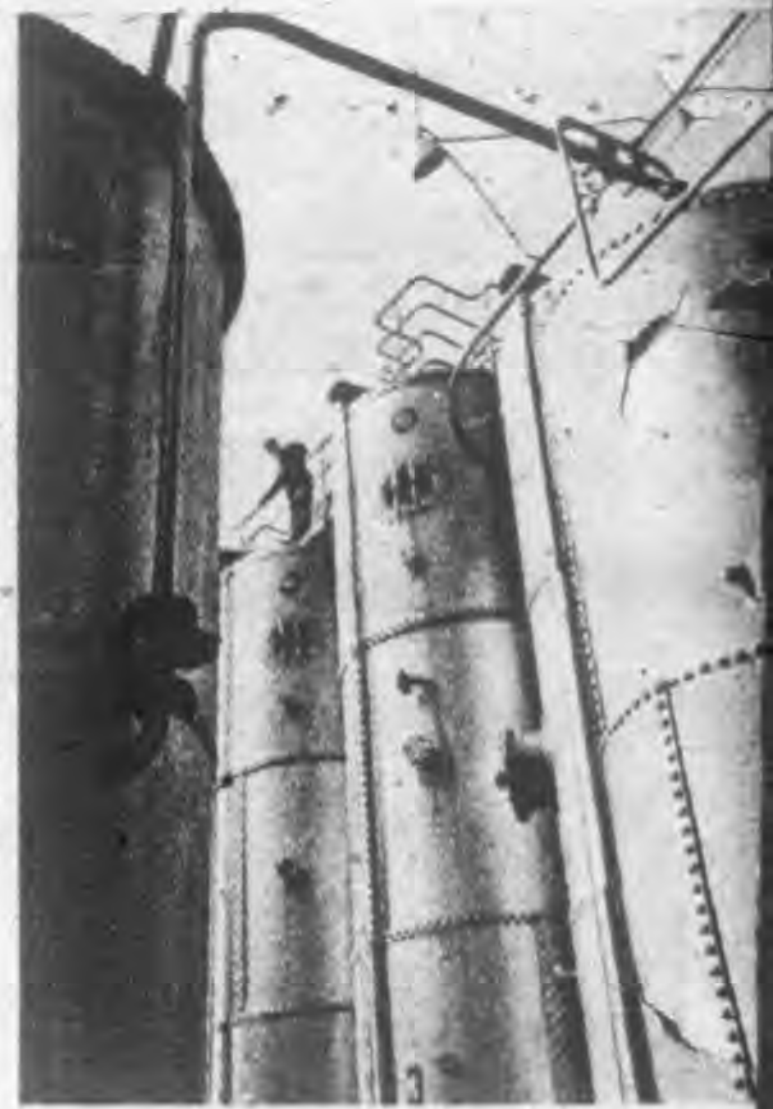
維分，蘇桶工人 ○雜用打中廠造 織以水成，絲 A forest of towers—the landmark of the factory which produces artificial silk. The high tanks are filled with soda-lye which breaks up the cellulose.
