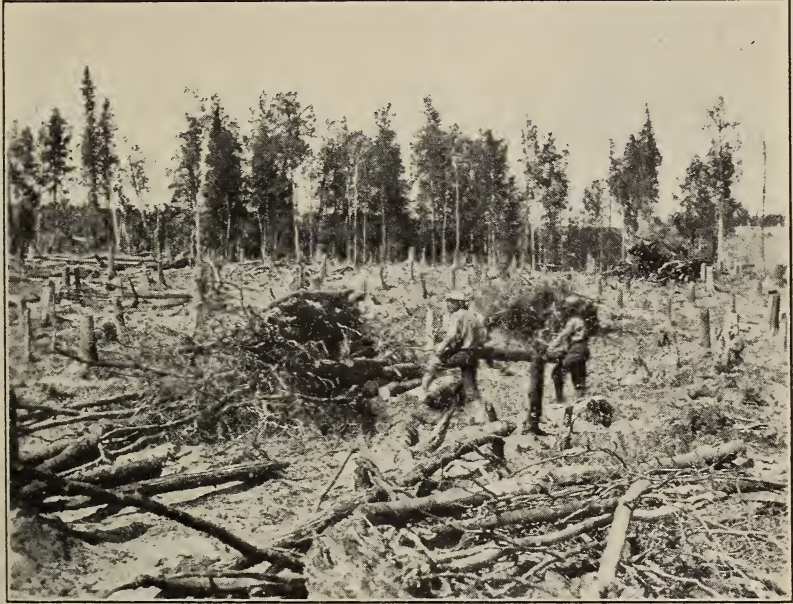
FIGURE 11.—Piling partly burned logs, Matanuska station
