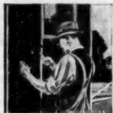
Applying Johns-Manville Housline
