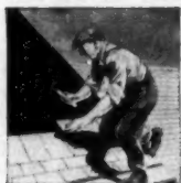
Applying Johns-Manville Asbestos Shingles
