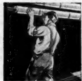
Applying Johns-Manville Improved Asbestocel
