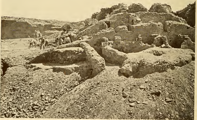
FIG. 73.—The outer southwest corner of Pueblo del Arroyo during the course of excavation. In this section, nine rooms, previously unsuspected, were discovered. (Photograph by O. C. Havens. Courtesy of the National Geographic Society.)
