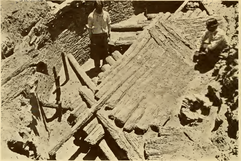
FIG. 69.—The roof of a Pueblo Bonito council chamber was a very complicated affair. Beginning on eight or ten low masonry supports, pairs of logs lay close to the kiva wall; above these were other poles laid in threes, fours, etc., until a neat vault, flat on top, covered the room. (Photograph by O. C. Havens. Courtesy of the National Geographic Society.)
