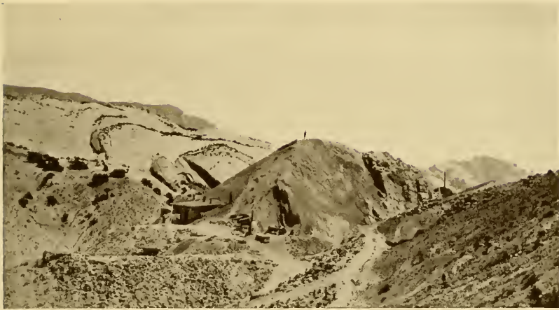
FIG. 17.—View of the quarry at the Dinosaur National Monument. The slope in the center foreground was excavated for dinosaur remains by the Carnegie Museum. The dump may be seen in the lower left hand corner. (Photograph by Earl Douglass.)
