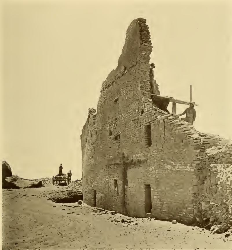
FIG. 71.—Extensive repairs have been made to strengthen the shattered walls of prehistoric Pueblo Bonito and preserve its masonry for future generations. Four stories are evident in this particular view. (Photograph by Neil M. Judd. Courtesy of the National Geographic Society.)
