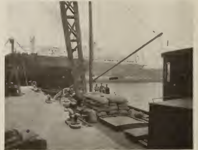
MARINE LEG UNLOADING BARGE
