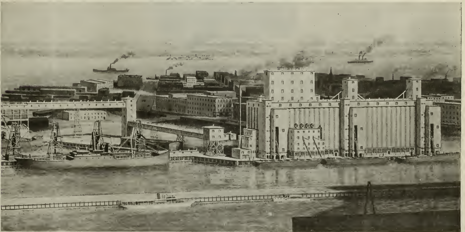
THE NEW YORK STATE ELEVATOR NOW UNDER CONSTRUCTION IN GOWANUS BAY, NEW YORK HARBOR
