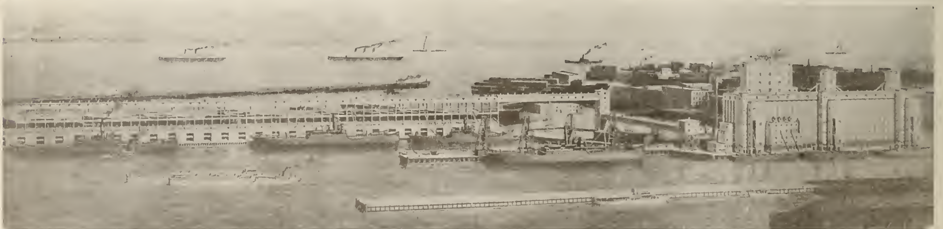
New York State Barge Canal Terminal Elevator Now Under Construction
