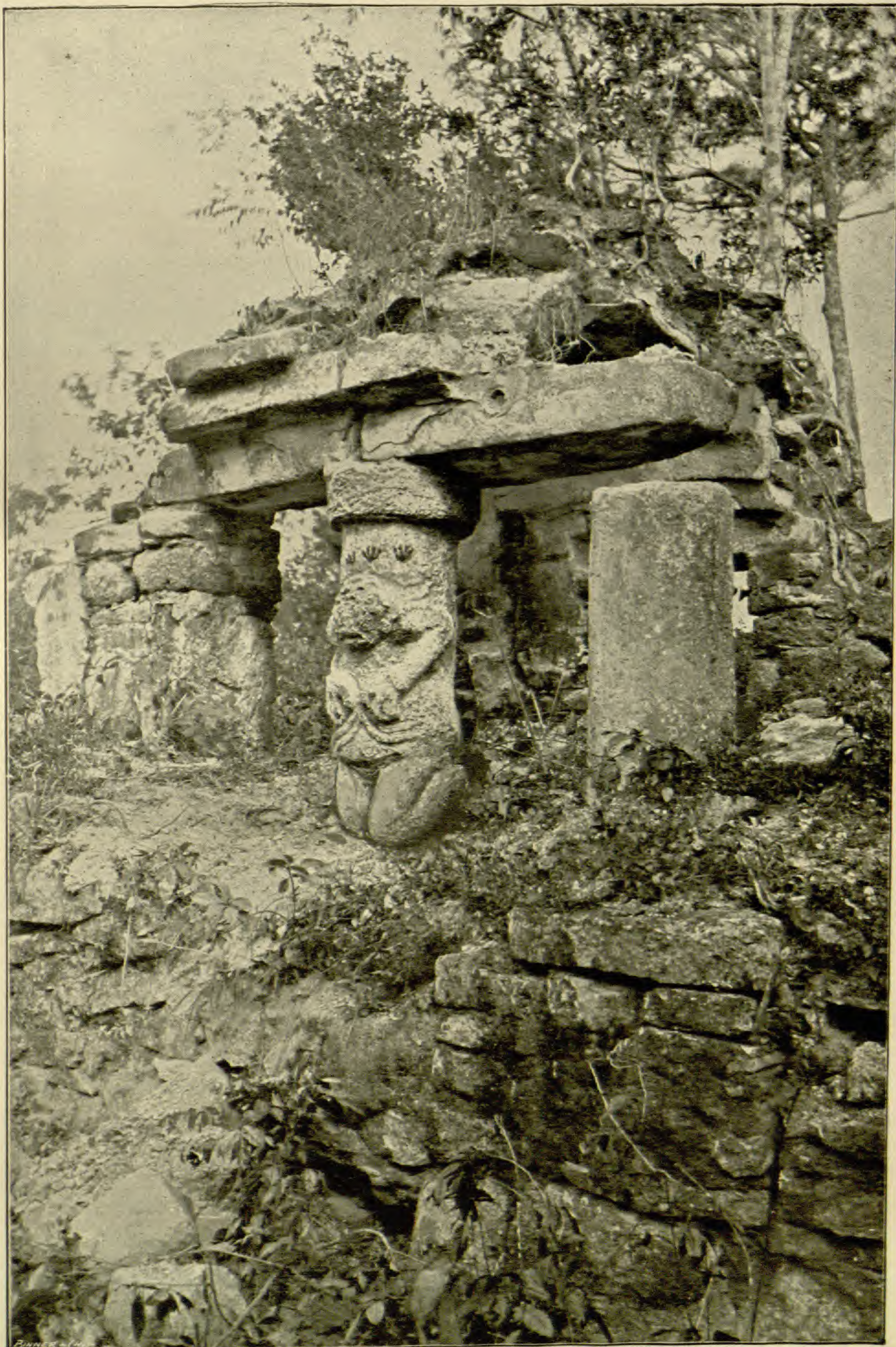
Fig. 4. Miniature portal of a small temple on the Island of Cozumel, a little entrance only 4 feet 6 inches high, to a diminutive building not over 20 feet square by 10 to 12 high resting on a terrace about 5 feet high, of the two round columns supporting the stone lintels, one is carved to represent a kneeling human figure. From a photograph by Mr. E. H. Thompson.
