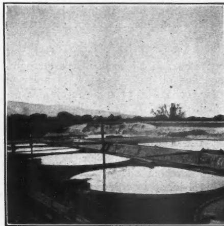
SAND TANKS NOW IN USE AT ANGUSTIAS MILL
