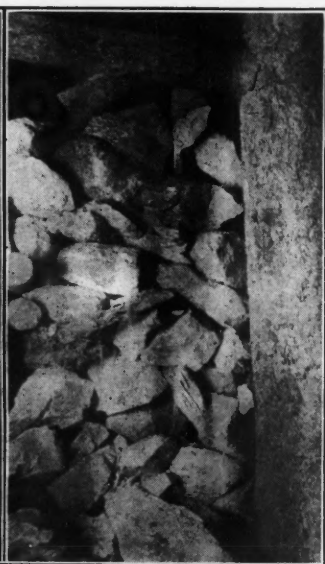
FIG. 3. ROCK FILLING BETWEEN CRIBS
