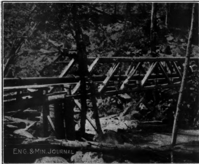
HIGH-PRESSURE PIPE TRESTLE, 600 FT. HEAD
