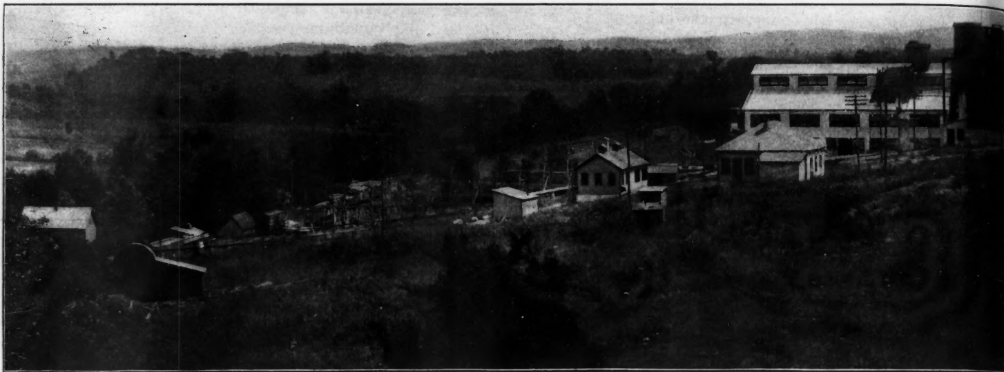
CONCENTRATOR BUILDING, AMERICAN ZINC CO. OF TENNESSEE, A SUBSIDIARY OF THE While designed to treat 1000 tons of ore per day, the actual capacity is from 1200 to 1400 tons per
