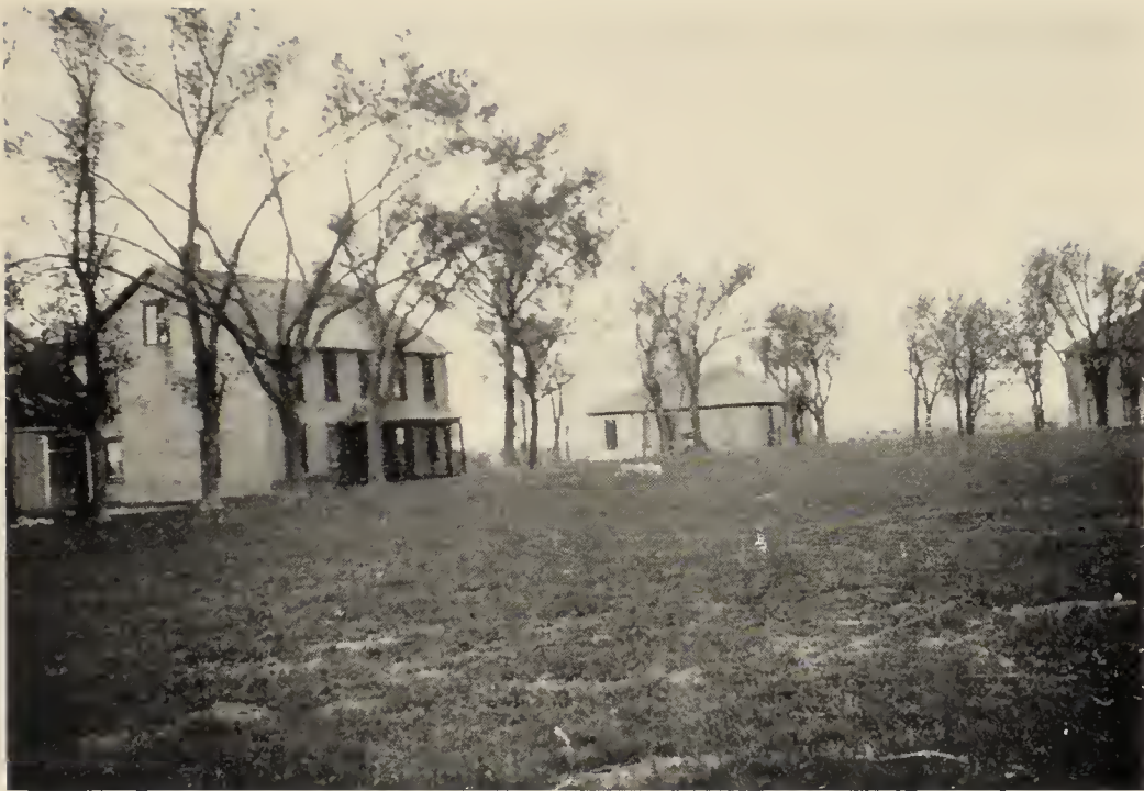
FIG. 23. Old Fort Sisseton, looking across the parade ground to the officers' quarters.
