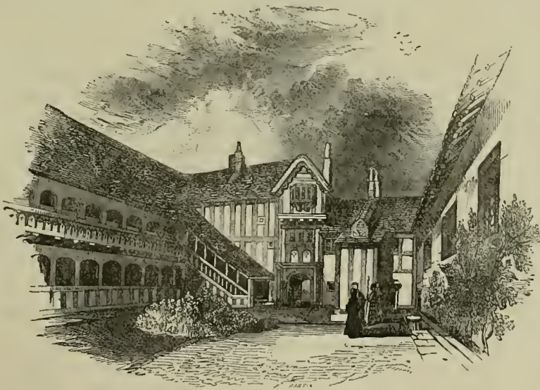
Leicester's Hospital, Warwick.
