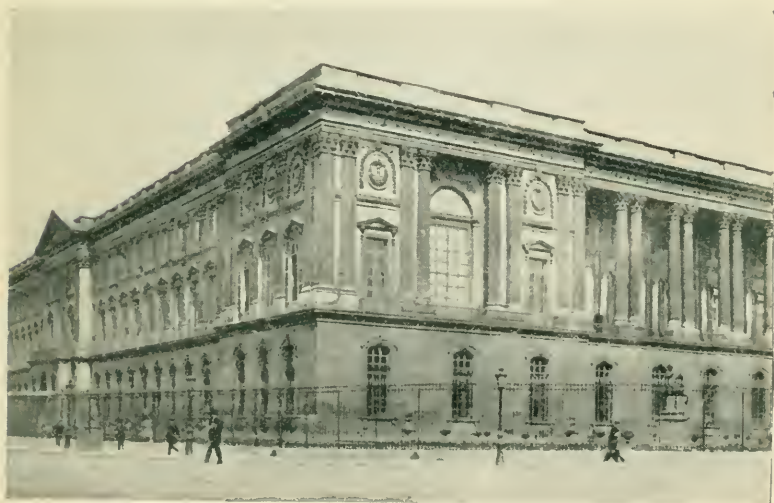
COLONNADE, EAST END OF LOUVRE, BUILT BY LOUIS XIV.
