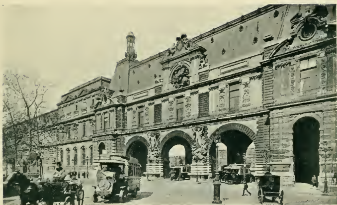
SECTION OF LOUVRE BEGUN BY HENRY IV, TO CONNECT THE EASTERN END OF THE LOUVRE WITH THE TUILERIES.
