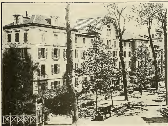
Hotel Des Sources, Hospital D, Macomb County Hospital
