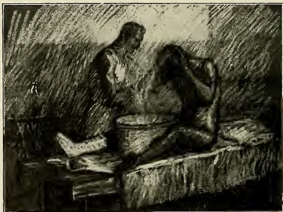
Removing Trench Mud.
