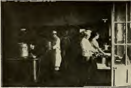
Kitchen at Hospital E
