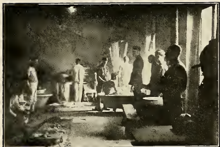
Receiving Room, Hospital B.
