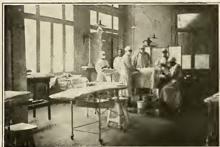
Operating Room, Hospital A.
