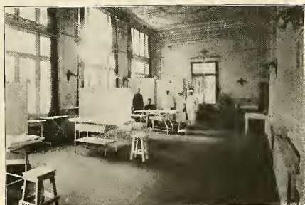
Operating Room, Hospital A.
