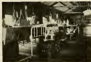
Interior of One of Our Shacks, Gun Hill Road.
