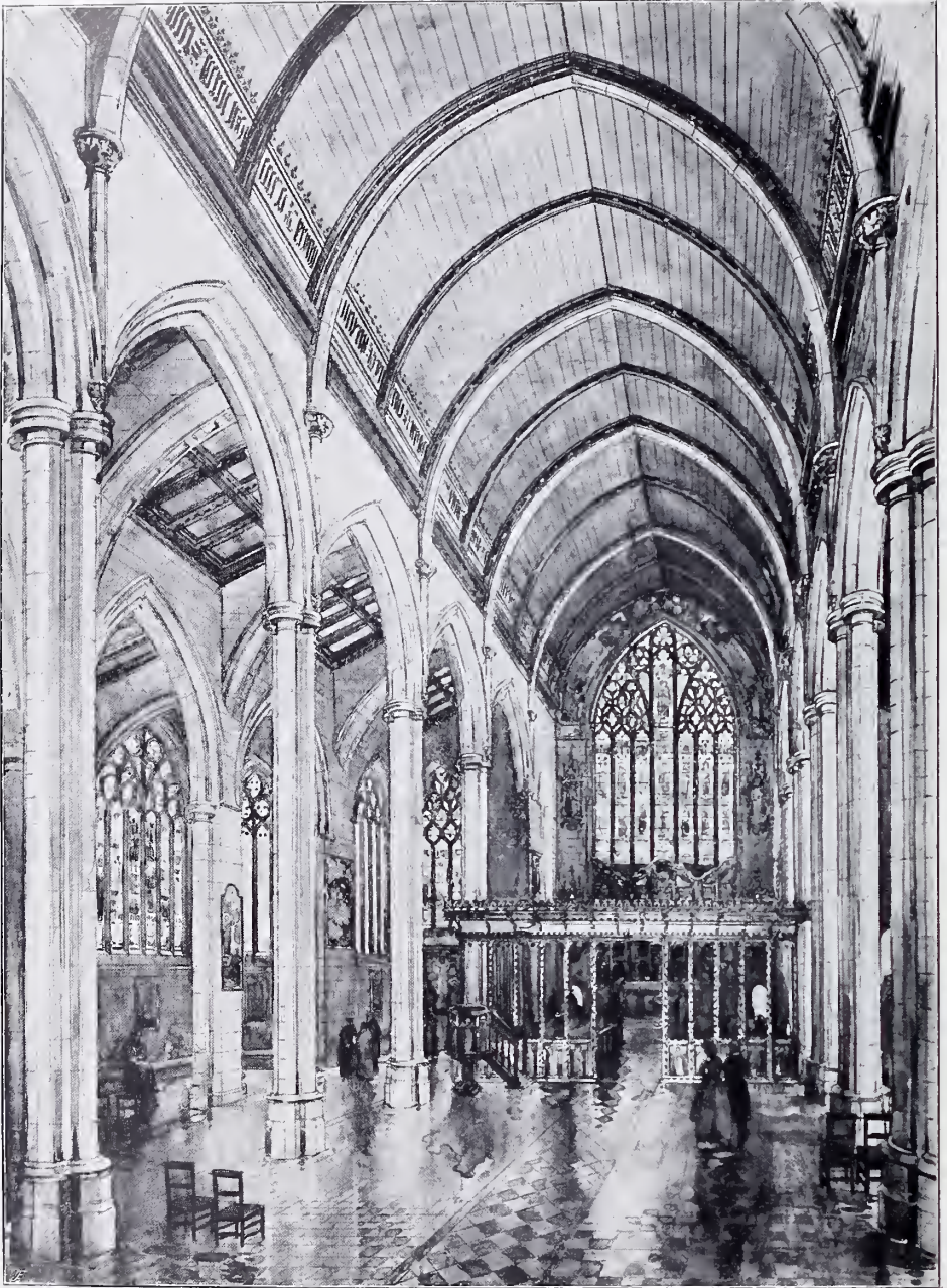
1657. Interior, New Church, Kensington, GEORGE F. BODLEY, A.R.A., Architect.
