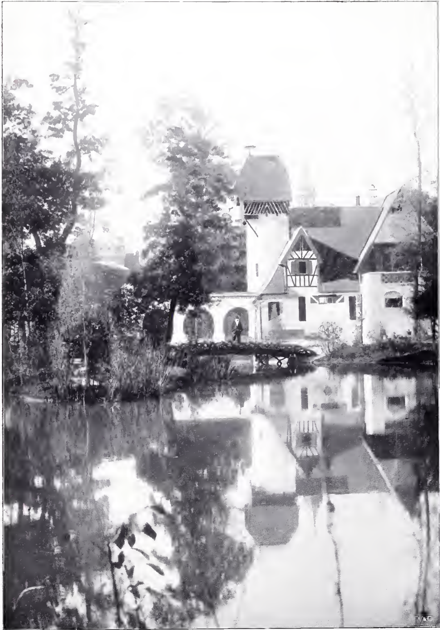
Stables, Villa Hauser, GEBR. RANK, Architects, Munich.
