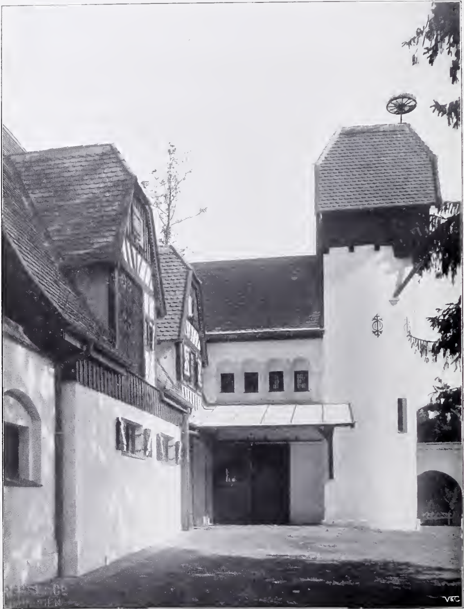
Stables, Villa Hauser, GEBR. RANK, Architects, Munich.
