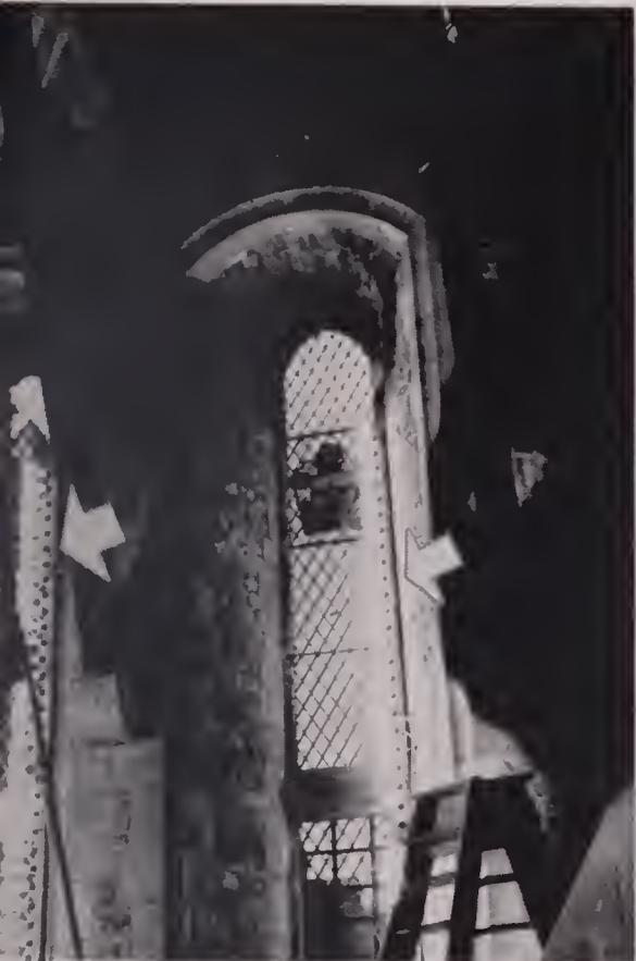
PHOTOFLOOD strip lights (arrows) mounted out of camera range in arches helped produce natural window glow in castle scenes.
