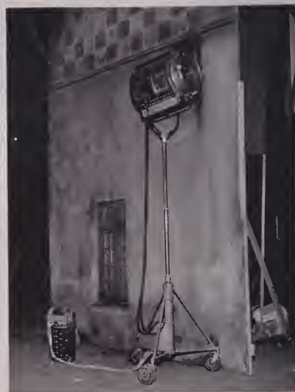
LAMP STAND at maximum elevation. Used chiefly for key and back lights, it affords quick changes in lamp position without need for erecting or reconstructing parallels.
