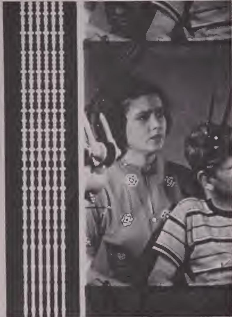
HALF 16MM. FRAME, above, shows six-unit sound track recently introduced by J. A. Maurer, Inc., makers of professional 16mm. cameras and sound recording equipment. All six tracks are identical, so that any lack of uniformity in the projector scanning beam will be minimized.
