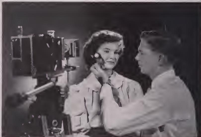
**THE LATITUDE** of color film is far less than that of black and white, and for this reason light meter readings should be taken carefully before starting to shoot. Basic light reading should be made for flesh tones, as shown here.
