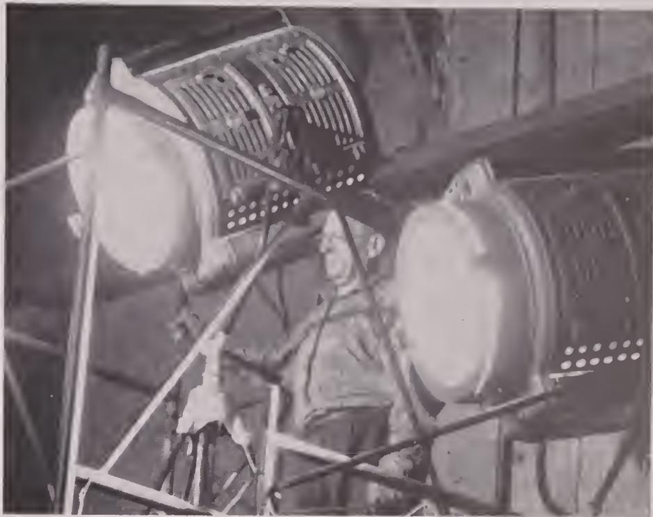
**USE OF powerful arc lamps** makes it possible to illuminate large sets with reasonable numbers of units and obtain desirable modeling effects and directional control over lighting. Moreover, color of the arc lamp light is ideal for color photography.
