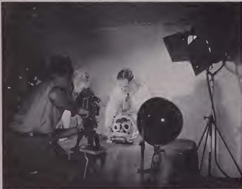
HERE a 16mm. industrial film is being photographed without sound, using a 16mm. Cine Special camera. The sound, in form of narration, sound effects and music will be post-recorded and combined with film later.
