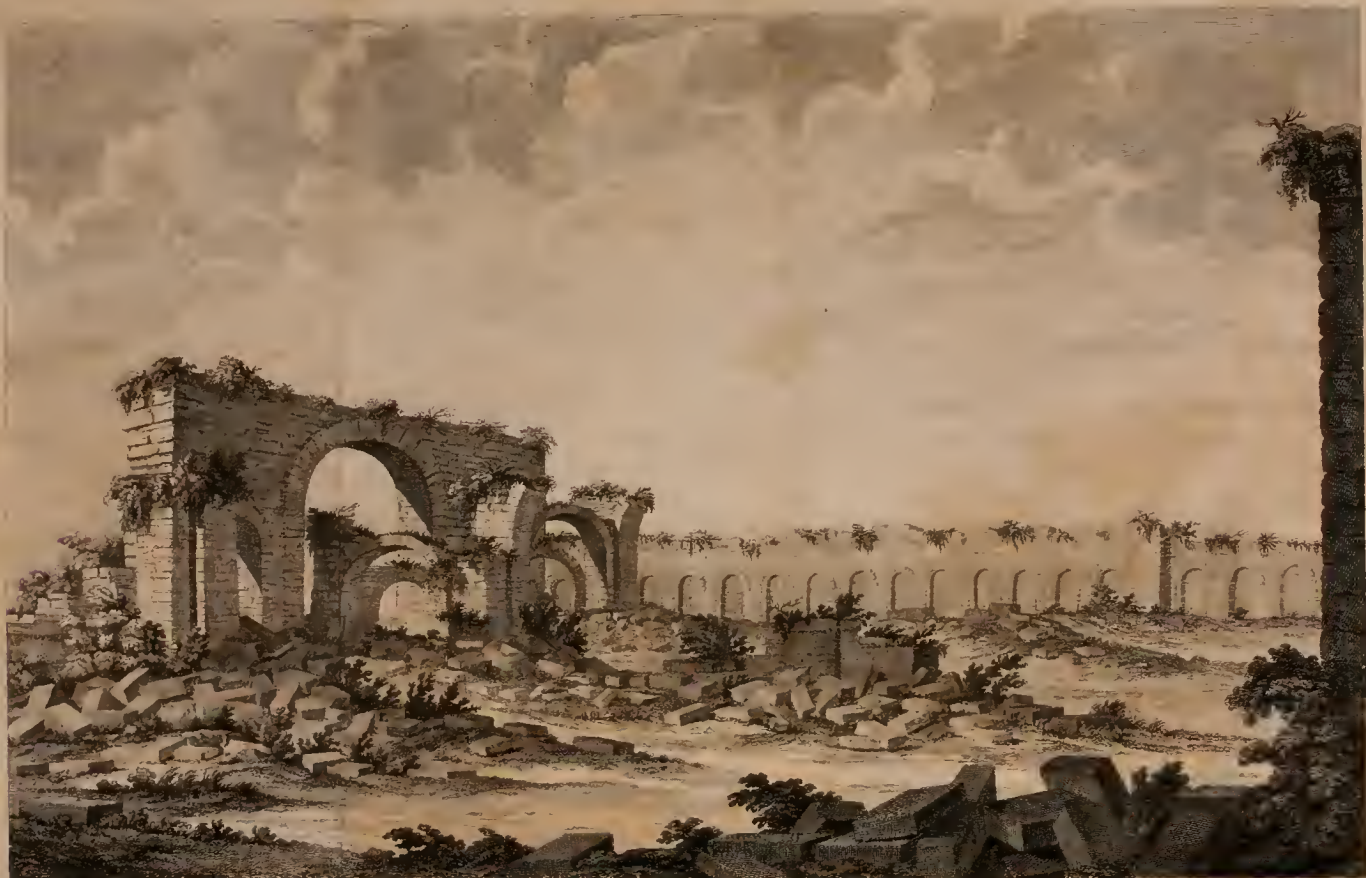
ANCIENT RUINS near TROY upon the ÆGEAN SEA. Supposed to be the work of ALEXANDER or LYSIMACHUS.
