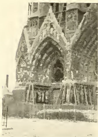
SUPPORTS TO RUINS AT RHEIMS CATHEDRAL.
