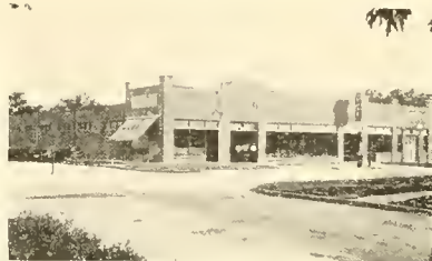
THE ROHWEDER GARAGE, PIPESTONE, WHERE THE RED CROSS BENEFIT DANCES WERE HELD
