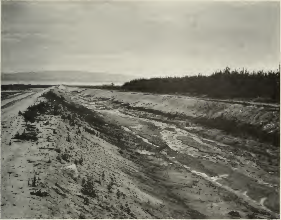
Fig. 3. View east of King Street canal following reconstruction (18 March 1978).
