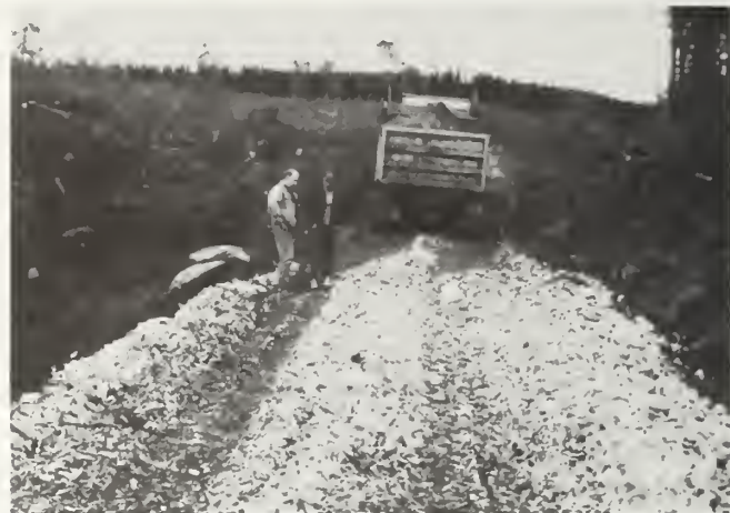
Figure 25.—Chunkwood added to stabilize a clay pocket.
