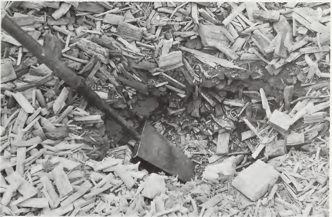
Figure 28.—Chunkwood particles permeated 6 inches into the clay road surface.
