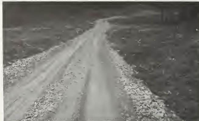
Figure 30.—Chunkwood road with native fill top grade.
