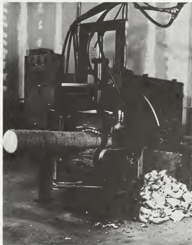
Figure 1.—Original laboratory model of the wood chunker (NCES, Houghton, Michigan).
