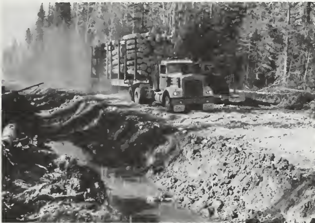
Figure 27.—Chunkwood road surface at Ft. Nelson, B.C., Canada.
