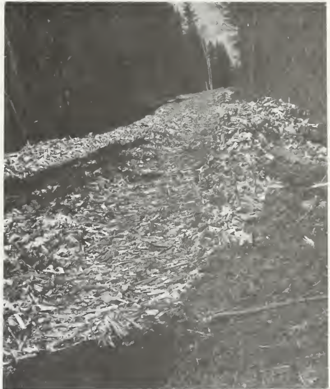
Figure 24.—Chunkwood road in Wisconsin.
