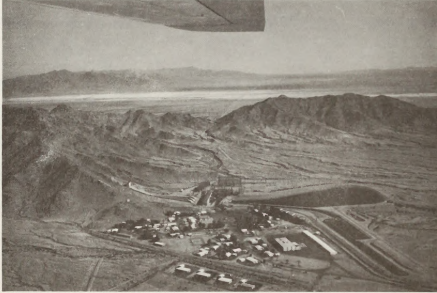
Figure 2.13 Iron Mountain Pumping Plant complex
