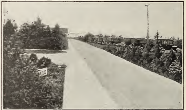
Entrance to office, display grounds and packing houses
