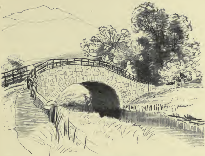
Bridge over the Bowmont Water.
