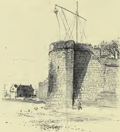
Walls of Berwick, low tide, showing storm drum.
