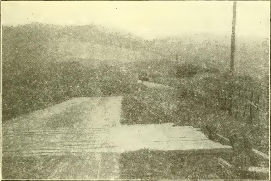
FIG. 181.—Horizontal Displacement During the San Francisco Earthquake shown by Road and Fence Line (see page 320).<sup>4</sup>
