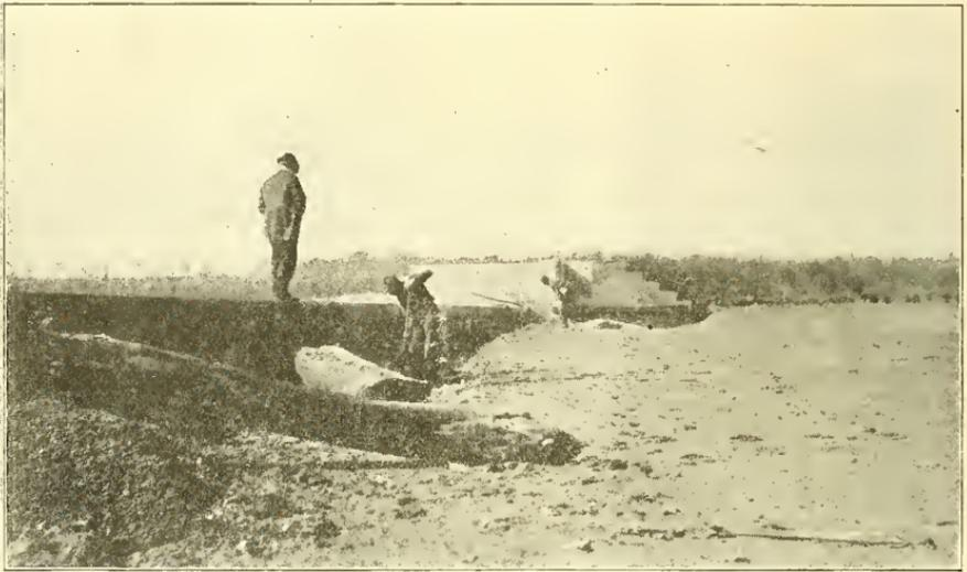
FIG. 182.—Deposits of Sand and Gravel behind the Danville Dam.
