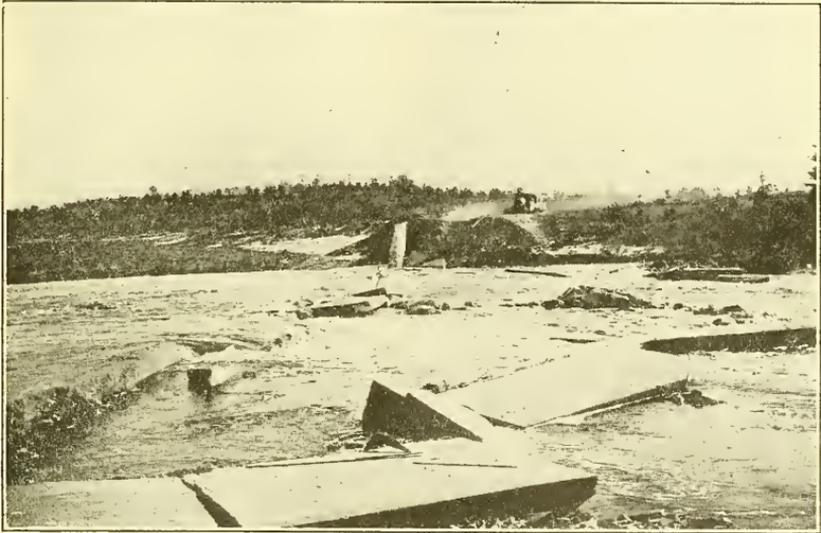
FIG. 323.—Break in Earth Embankment at Hatfield Dam.
