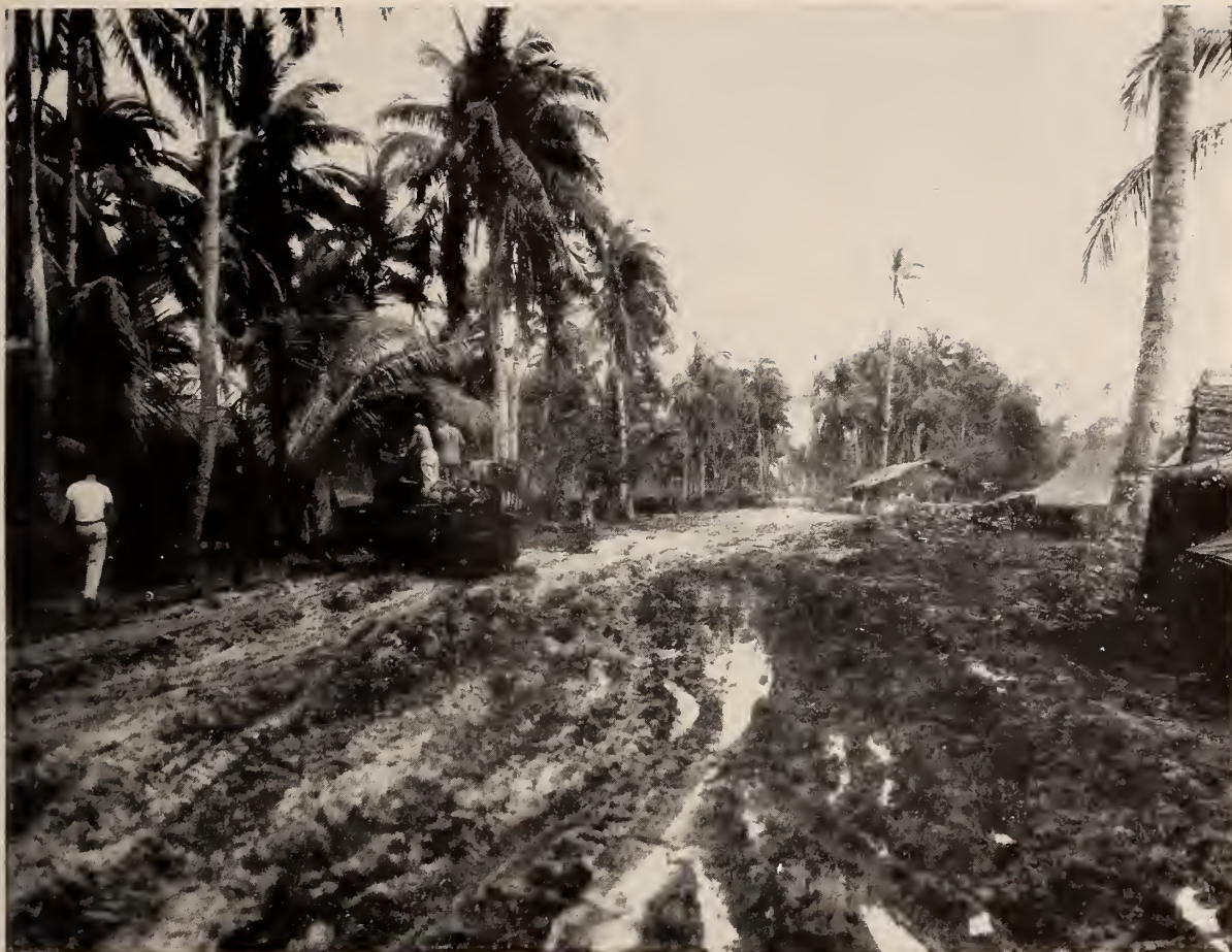
MUD AND RAIN constituted formidable obstacles, delaying troop movements and greatly impeding airstrip construction. This was the living area of Marine night fighter pilots first to land on Leyte.
