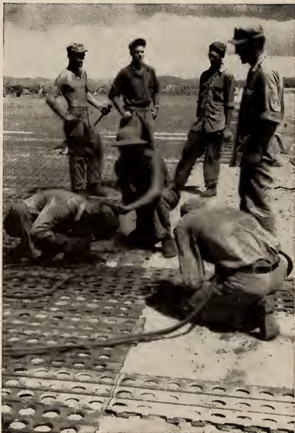
ARMY ENGINEERS work fast to get Tacloban's steel matting laid before arrival of Fifth Air Force P-38's to take over air support over Leyte, 27 October 1944.
