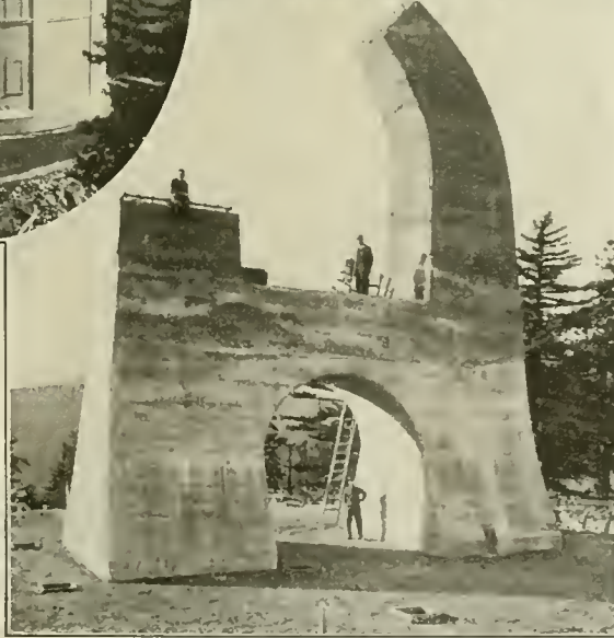
Above: The building complete, up to the covering of the dome. This is furnished with a system of shutters which with the double wall permit an even temperature to be maintained in the interior of the building
