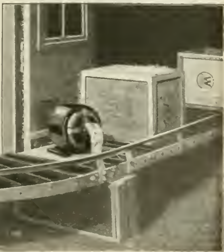
By means of curves, switches and other appliances the conveyers may be run around corners, partitions and over floors
