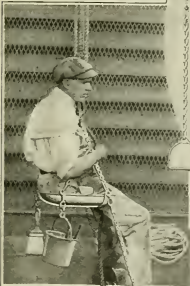
Short chains to hold pots and brushes depend from the back of the seat
