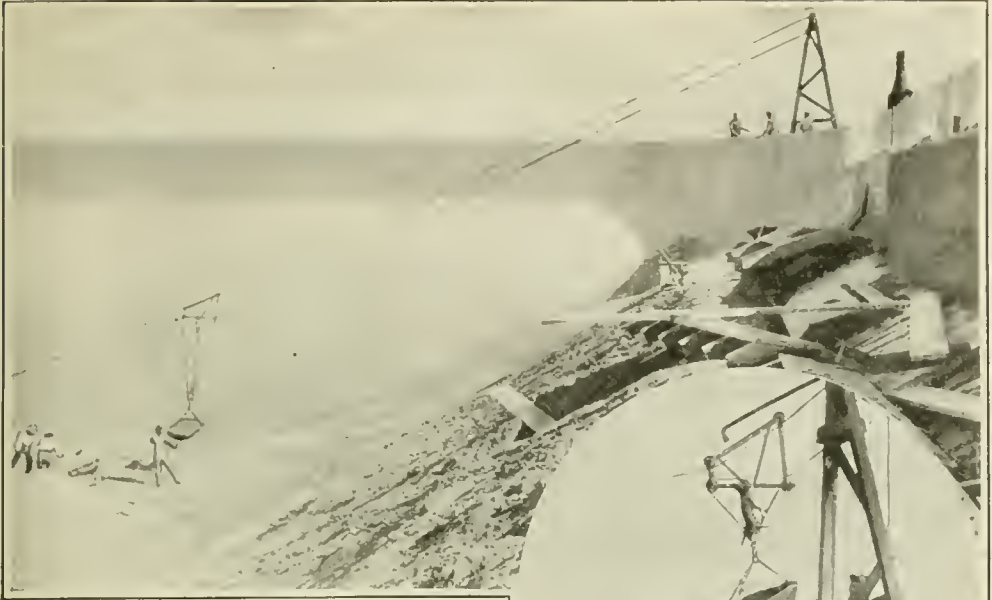
How the Stone and Old Concrete Were Removed from the Basin by the Improved Cableway
