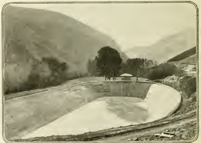
By lining a useless old pond with concrete five million gallons were added to the city's storage water supply
