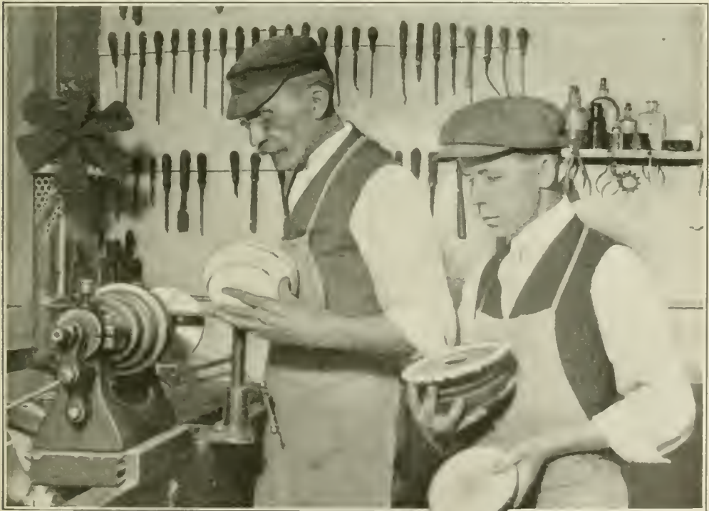
A Good Workman Can Cut the Forms of Perhaps Two Dozen Pipes from the Raw Material in a Single Working Day. These Forms Only Rudely Resemble the Ultimate Pipe shape
