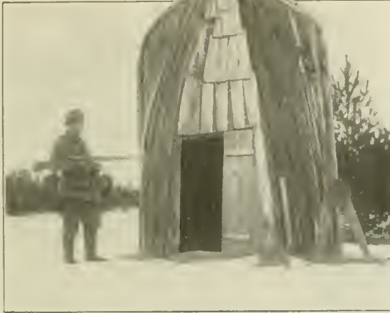
The sentinel's hut made out of the keel of a discarded boat. When made watertight by patching and filling the gaps it made a comfortable enough shelter
