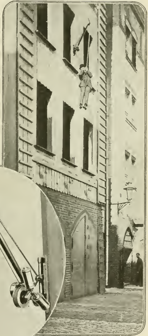
To escape from a burning building, a belt is put on, a safety-hook is adjusted and a swift descent is made through space
