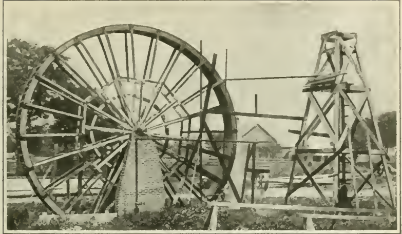
Electric current enough is generated by this plant, run by an artesian well, to operate a farm-mill, feed-chopper, lathe and other machinery used on the farm
