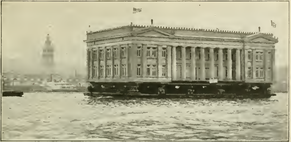
The spectacle of this one thousand-ton Exposition building floating serenely down San Francisco Bay caused residents of the Coast to doubt the testimony of their own eyes
