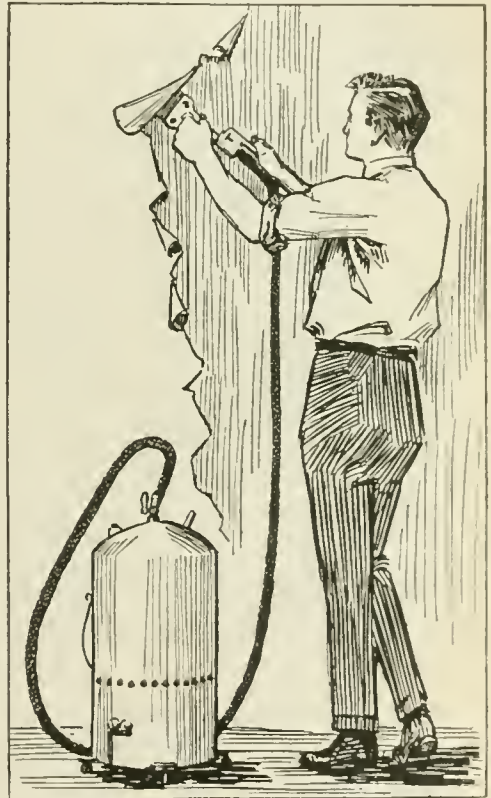
Every bit of wallpaper should be removed before beginning the work of repapering
