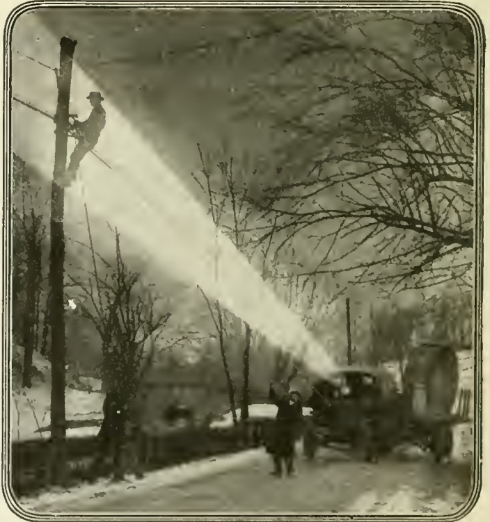
The telephone lineman making a quick repair under the beam of a searchlight which is mounted on an emergency truck
