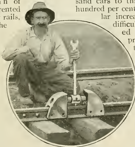
One of the clamps fits over each rail-end and a screw-rod spreads or joins them
