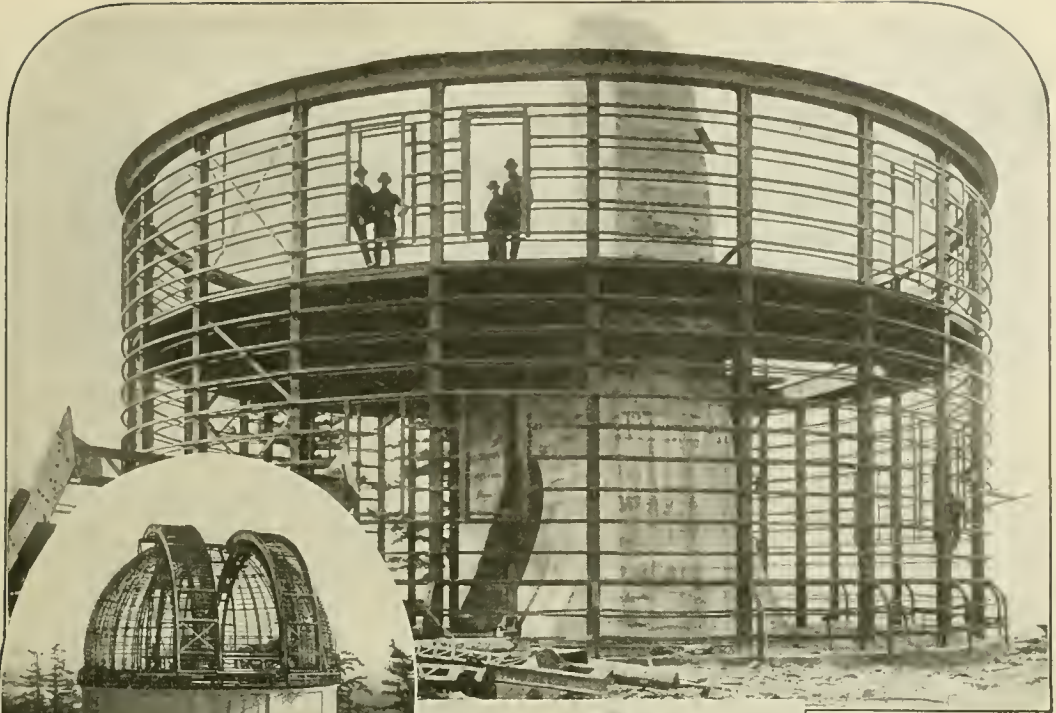
Above: The iron framework of the walls. Horizontal ribs are attached in pairs both to the outer and inner edges of the upright beams, thus forming a double wall with an intermediate air-space
