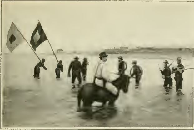
Signal detachment, with flags and telephones, fording a river to lay a line of communications
