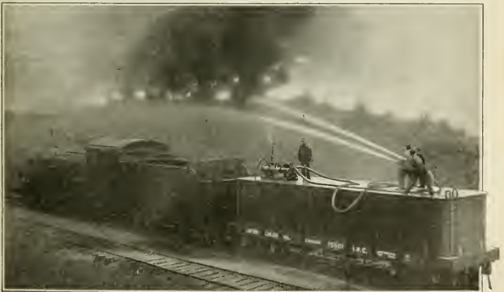
The fire-fighting apparatus is kept under steam so that it can be quickly transferred to any point on the railroad's system where fire may be threatening property worth millions
