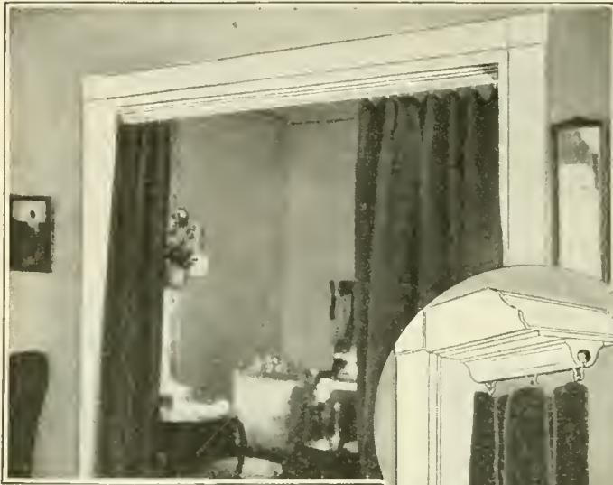
Wooden Balls Attached to Metal Hooks Which Receive the Curtain Rings Slide in a Hidden Groove with the Movement of the Curtain
