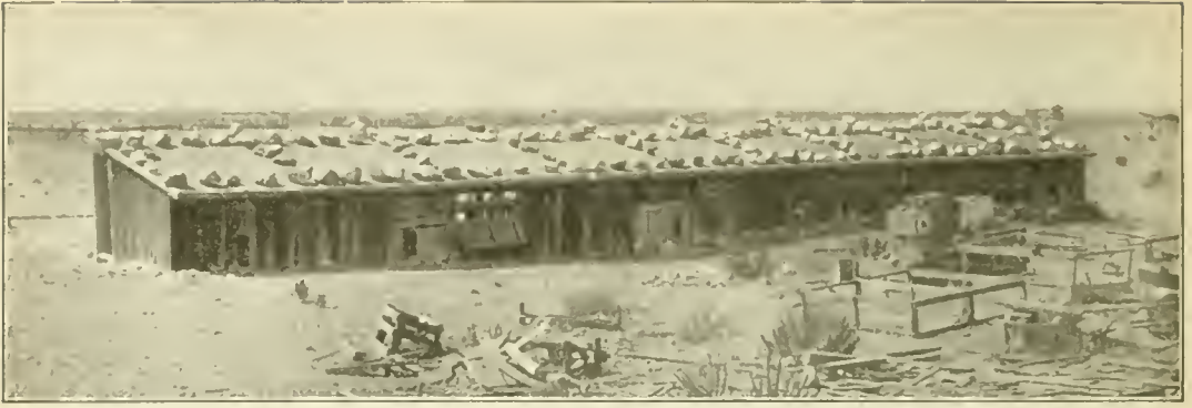
Several tons of stones were used to insure the safety of these henhouses. Care was taken to place the stones directly above the roof supports of the partitions to prevent sagging
