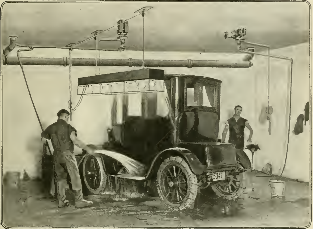
A flood of light may be thrown upon any portion of the body of the automobile without subjecting the bulbs to contact with the spray. The box can be elevated to any height
