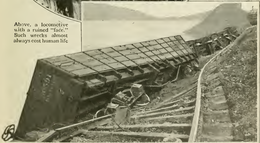
A slip and slide into the river is all that happened here, but it took a complete track-laying gang in addition to the wrecking-crew to get the line open again and restore train schedules
