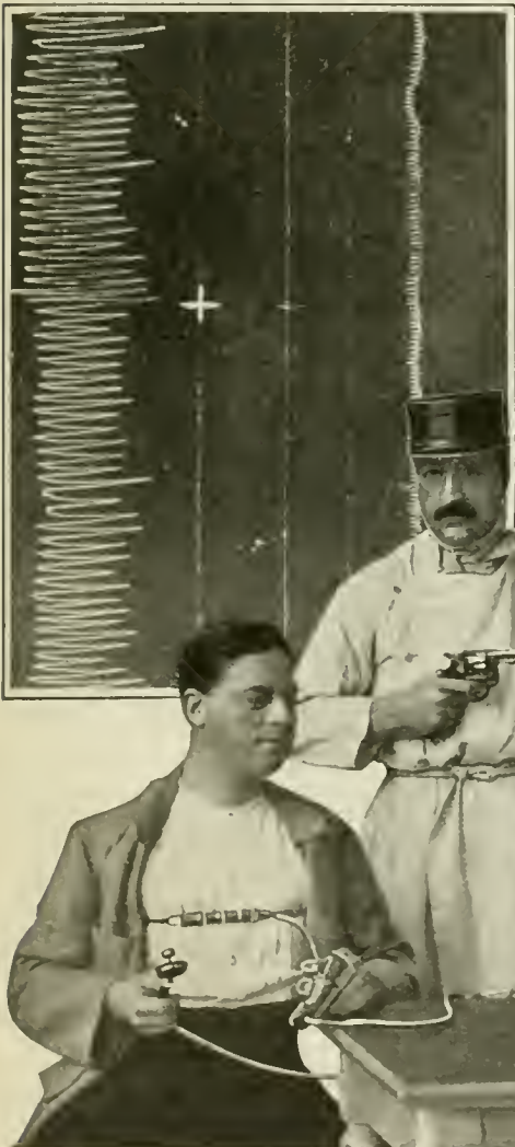
The d'Arsonval chronometer which records on a smoked paper cylinder the pulse-beats, respiration and nervous tremors of the applicant when a pistol is fired behind him
