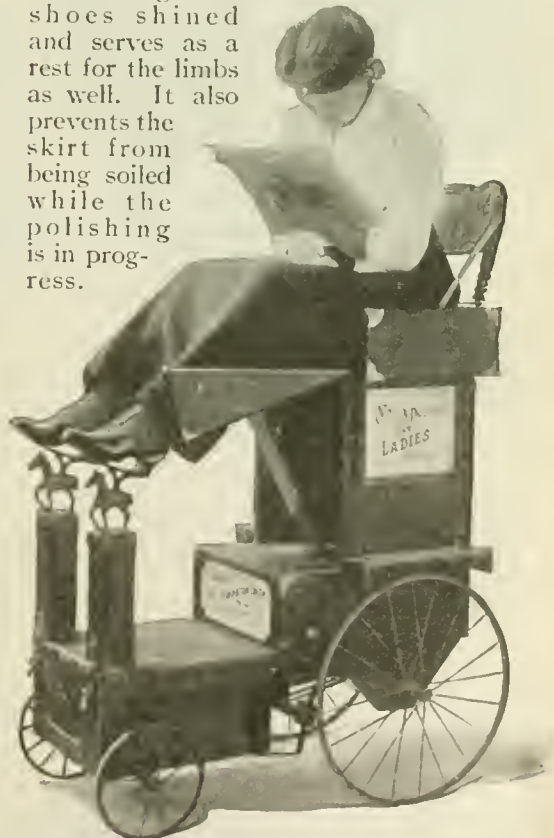
The Wooden Tray Is Adjusted by a Slight Movement and Serves as a Rest for the Legs and a Protection to the Skirts
