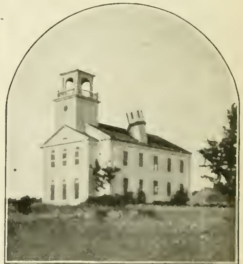
The spire was blown off the steeple and its sharp end pierced the roof and stuck
