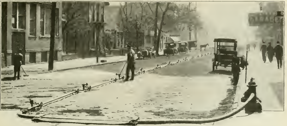
A man with a wrench opens the nozzles in succession, each stream cleaning to a line ahead of the next nozzle until the operator has gone over the entire area between hydrants
