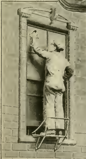
Below: A window-cleaning chair of solid steel, with a firmly-clamped seat of heavy wood
