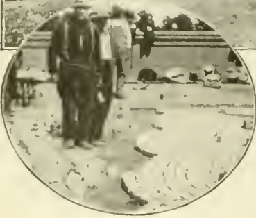
The new type of granite block pavement is laid in concentric interlocking rows, called the oyster-shell pattern
