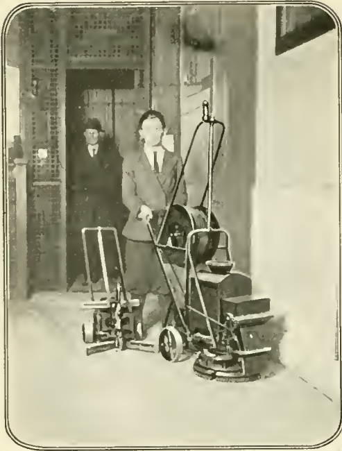
The machine is fitted with four to eight brushes the pressure on which is regulated
