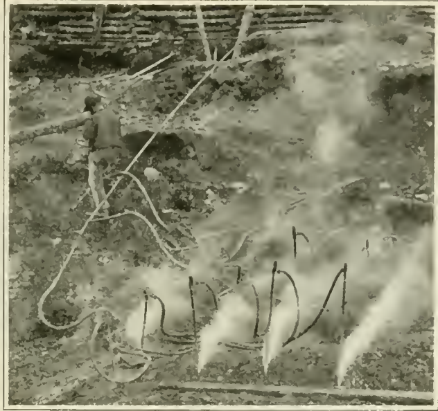
Long, hollow tubes are driven into the ground in rows and steam is forced through them for several hours
