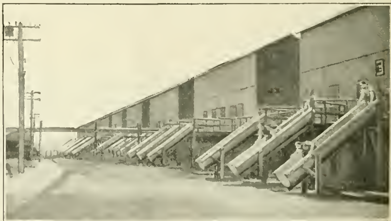
The Workmen Run for the Windows, Leap Into the Chutes and Slide Gently to the Ground in the Fraction of a Minute
