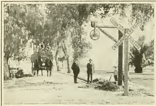
The automatic flagman at a crossing. At right, detail of four different installations
