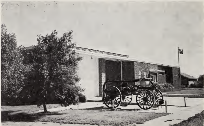
Public services originate from modern, well equipped structures such as this fire hall
