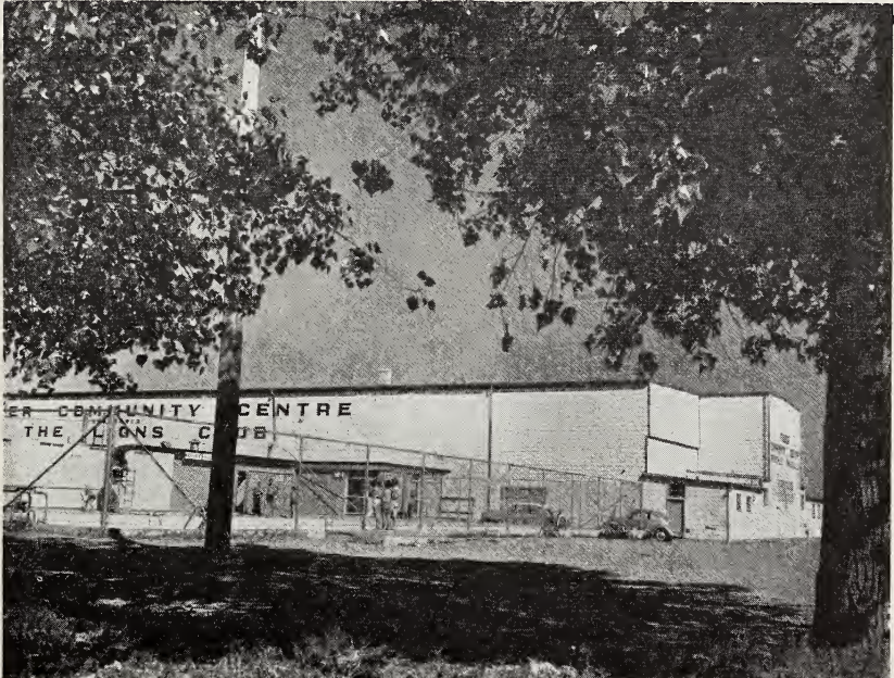
Taber's Community Center includes a swimming pool
