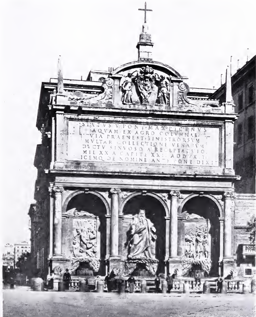
Fontana dell' Acqua Felice, Rome, about 1590 Designed by Domenico Fontana
