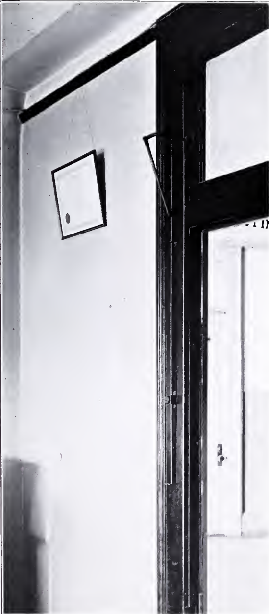
Moore Building, San Antonio. These partitions, though 18 years old, are absolutely free from cracks. 27 gauge Kno-Burn with channels 12" o.c. was used.
