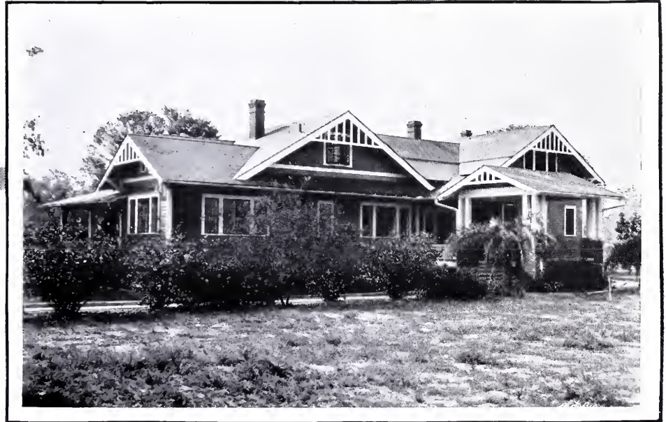
Home of Miss K. Jackson, Tampa, Fla.; Architect, F. J. Kennard, Tampa; Contractor, J. S. Sweet, Tampa Covered with Carey Asfaltslate Shingles
