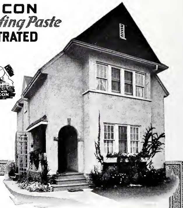
Waterproofing was used in this Stucco
