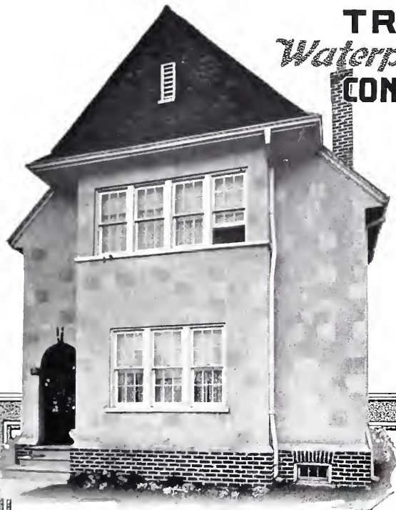
No Waterproofing used in this Stucco
