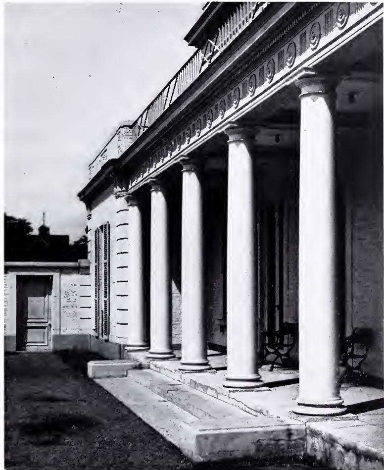
Detail of Forecourt Entrance, House of Benjamin Nields, Esq.
