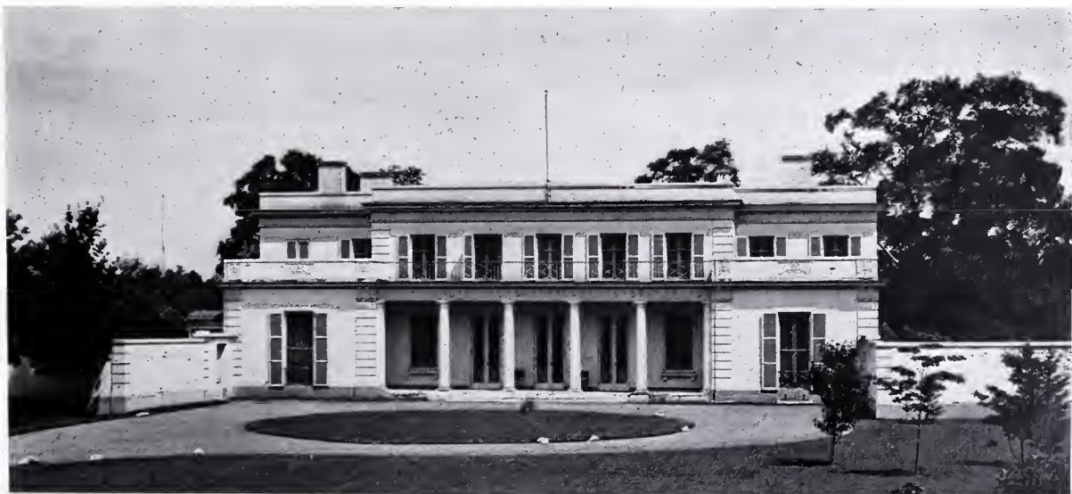
View of Main Facade on Forecourt, House of Benjamin Nields, Esq., Rye, N. Y.
