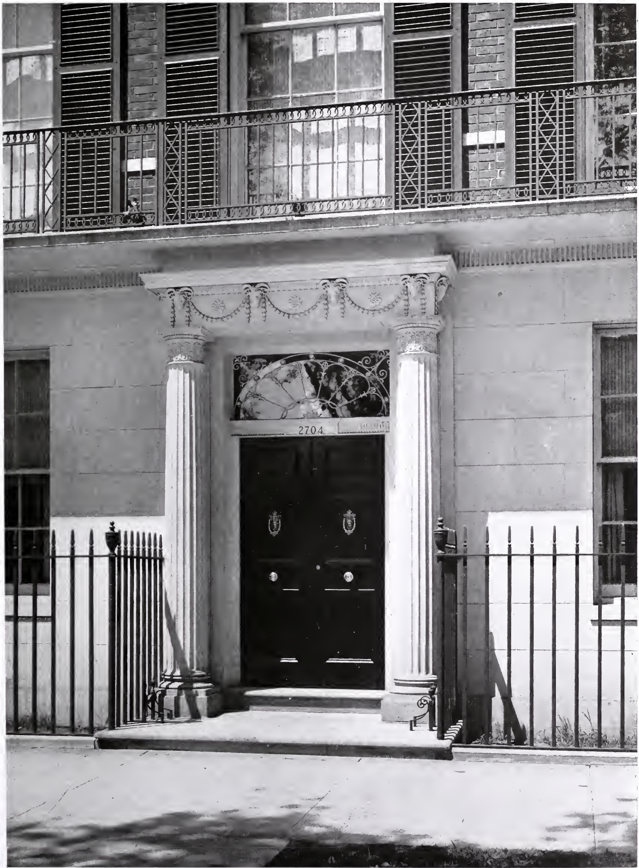
DETAIL OF ENTRANCE
