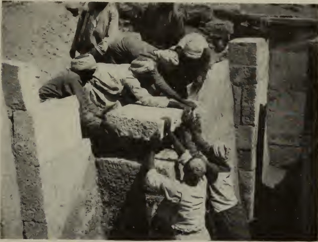
FIG. 20. REMOVING BLOCKS FROM FAÇADE
