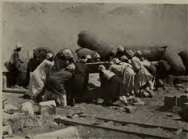
FIG. 18. PACKING LINTEL OF MAIN DOORWAY
