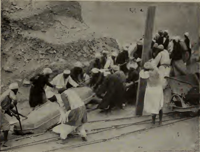
FIG. 17. HAULING LINTEL OF MAIN DOORWAY
