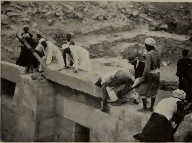
FIG. 16. REMOVING LINTEL OF MAIN DOORWAY
