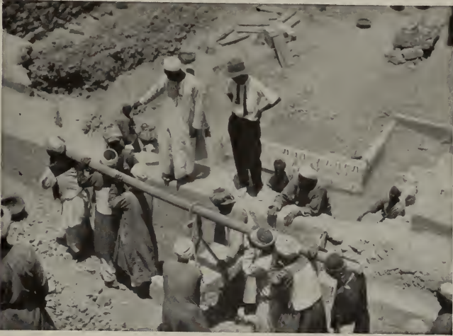
FIG. 23. METHOD OF CARRYING BLOCKS
