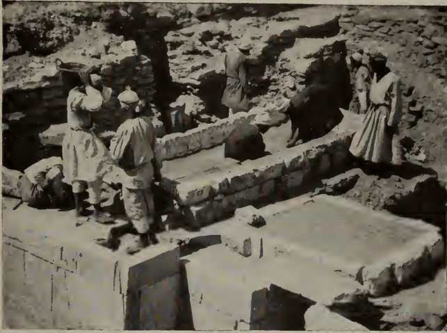
FIG. 15. PREPARING TO REMOVE UPPER COURSES OF DECORATED CHAMBERS, WHICH ARE FILLED WITH SAND TO PREVENT THE COLLAPSE OF THEIR WALLS
