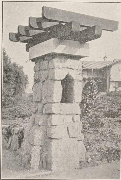
A street monument made of sandstone, redwood timbers and originality C. W. Leffingwell, San Rafael Heights
