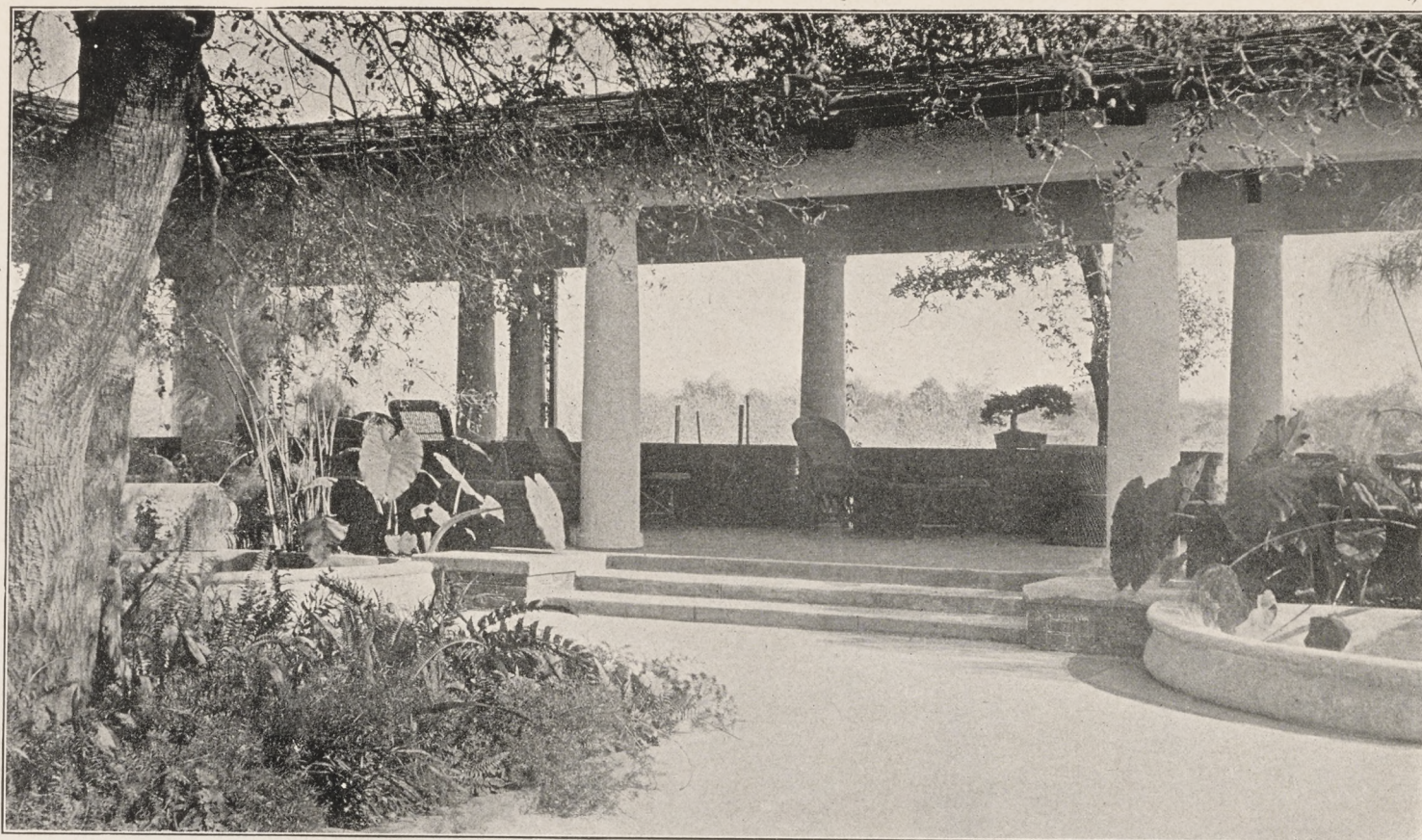
Unique Portico At Home of Gilbert Perkins—Myron Hunt and Elmer Grey, Architects
