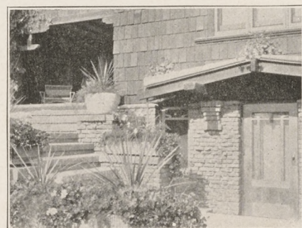
It is just such original bits as this basement entrance that is making the architecture of Southern California famous
