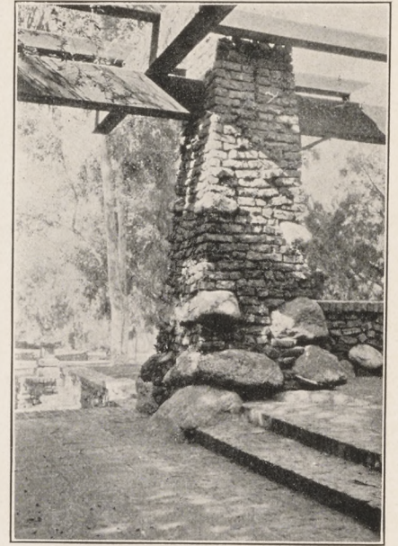
A wonderfully effective jumble of klinker brick, cobblestones and rough redwood timbers is found in the makeup of this pergola
