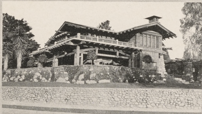
An Elegant and Elaborate Arrangement and Combination of Redwood Timbers, Malthead, Red-Brick and Cobblestones.
