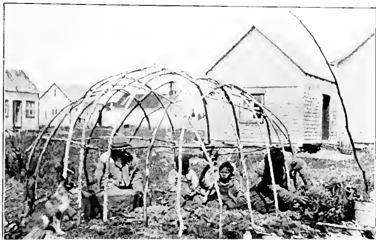
WIGWAM IN PROCESS OF CONSTRUCTION AT MINGAN.
