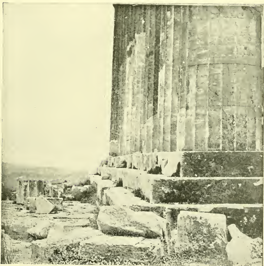
ILLUSTRATIONS SHOWING THE CURVES OF THE STYLOBATE OF THE PARTHENON. From photographs.
