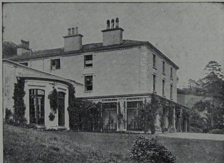
View of College from South-West
