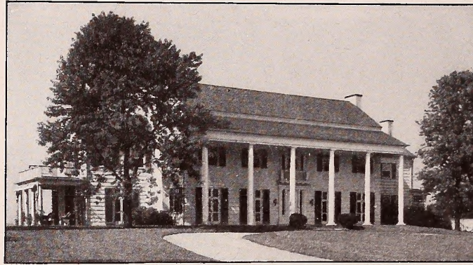
Shingled Walls and Brick Chimneys finished with Cabot's Old Virginia White John Russell Pope, Architect, New York
