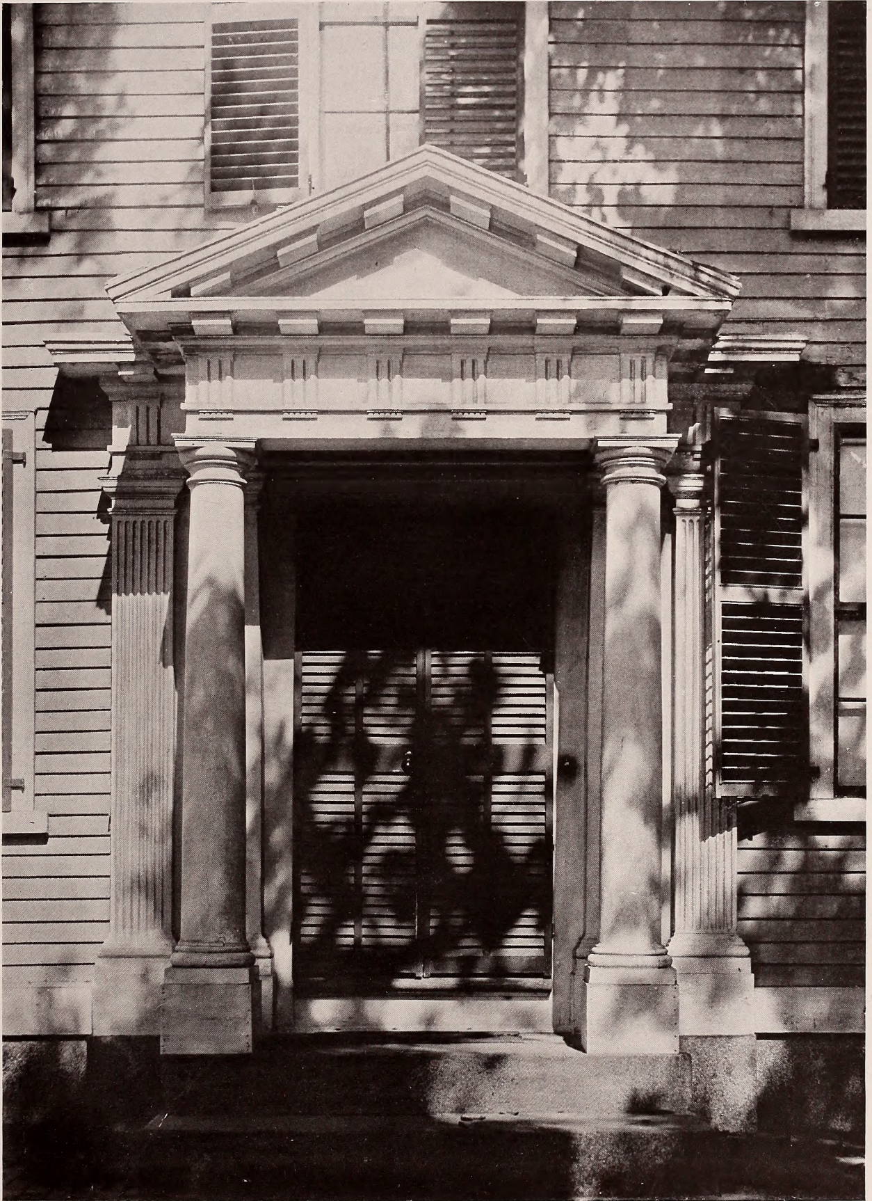
STEARNS DOORWAY, 384 ESSEX STREET, SALEM, MASS., 1785
