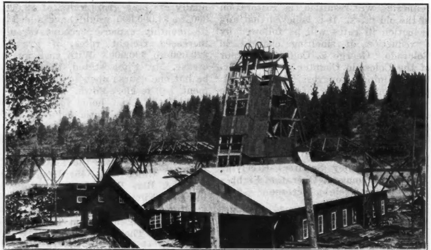
PLANT OF IDAHO-MARYLAND MINES CO., GRASS VALLEY, CAL., SHOWING HEADFRAME AND SHOPS
