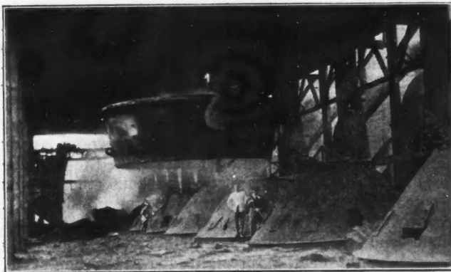
INTERIOR OF SINTERING PLANT, SHOWING POT AND SINTER GOING TO BREAKING FLOOR
