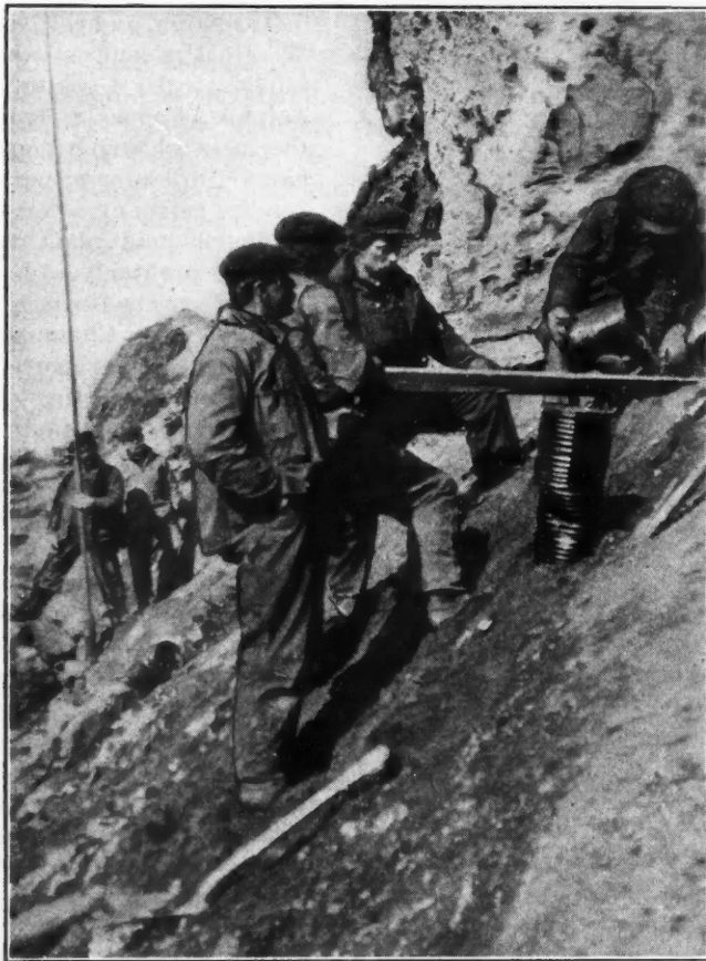
LOADING BLACK POWDER INTO "GOPHER HOLES"
