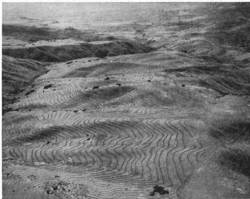
Figure 4.—Restoring an overgrazed semiarid range by contour furrowing. These furrows for holding moisture were installed on an Idaho range with the help of C.C.C. labor.
