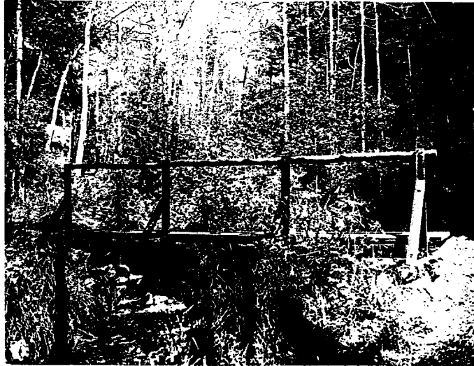
Photo No. 23 Example of foot bridge used extensively in Humboldt campgrounds.
