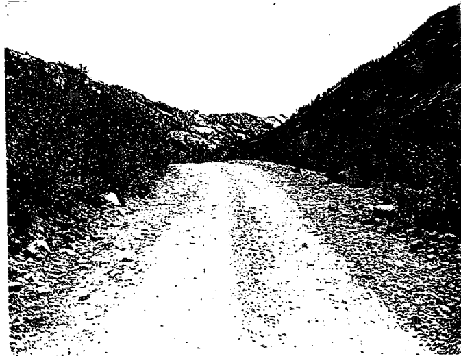
Photo No. 9 F.R. 21 in Lambille Canyon Showing condition of the road surface.
