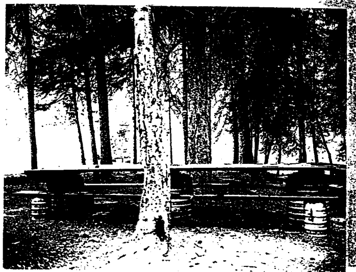
Photo No. 20 Permanent type of picnic table with poured concrete base.
