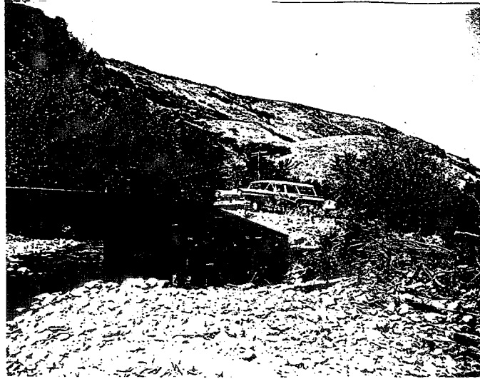
Photo No. 5 Bluster Bridge Showing erosion around wing wall.
