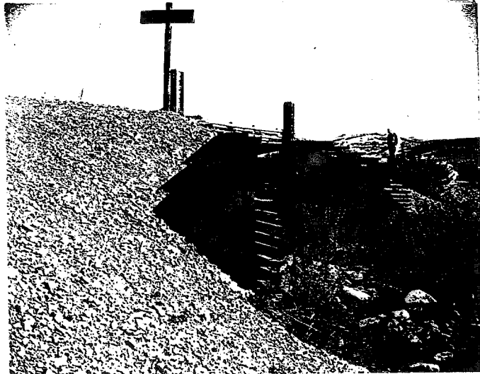
Photo No. 3 Martin Creek Bridge No. 1 Showing lack of fill behind wing wall.
