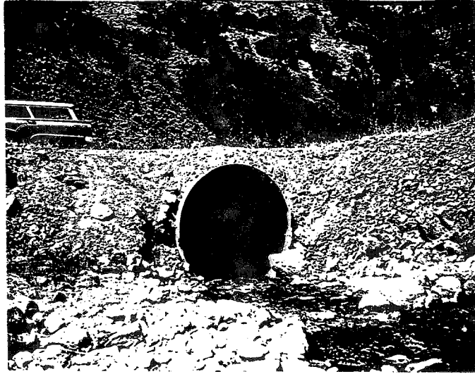
Photo No. 1 Jack Creek Culvert Showing limited depth of fill.
