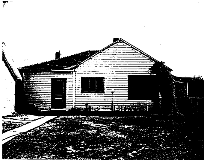
Photo No. 21 Side view of Gold Creek Ranger Station illustrating "add-on" type of construction.
