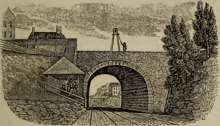
Arch over the Railroad, Bordentown.
