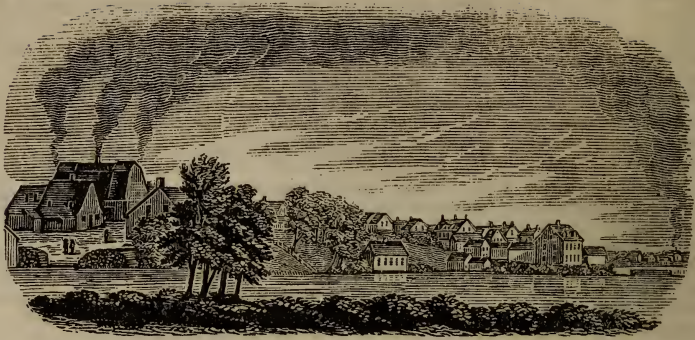
Northwest View of Millville.
