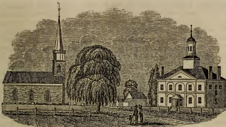
View of the Courthouse and Church, Hackensack.
