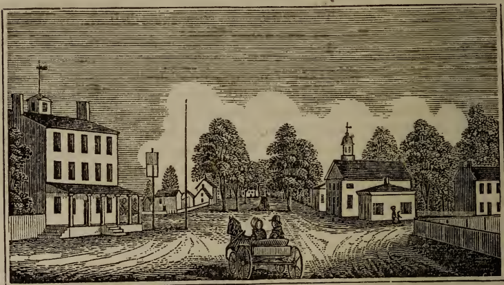
View of the County Buildings, May's Landing.
