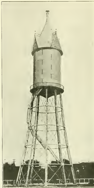
LARGEST WATER TOWER IN THE COUNTRY— JACKSONVILLE, FLA.
