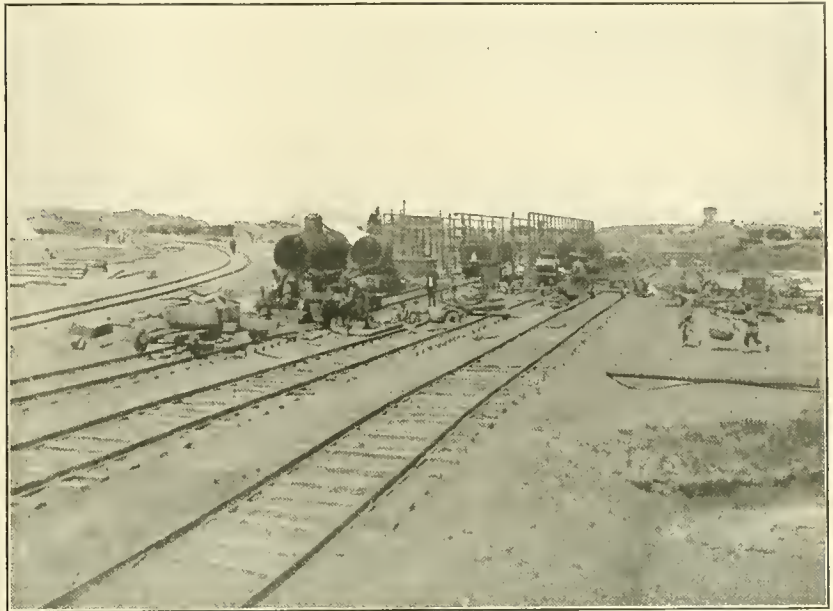
ERECTING BALDWIN COMPOUNDS AT VICTORIA BAY FOR CHINESE EASTERN RAILWAY.
