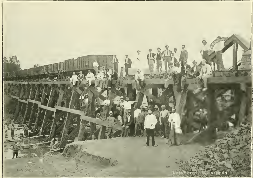
FIRST TRAIN OVER TEMPORARY TRESTLE.
