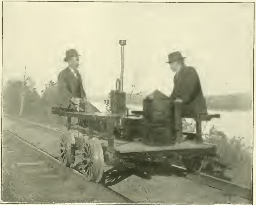
ELECTRICALLY DRIVEN INSPECTION CAR.
