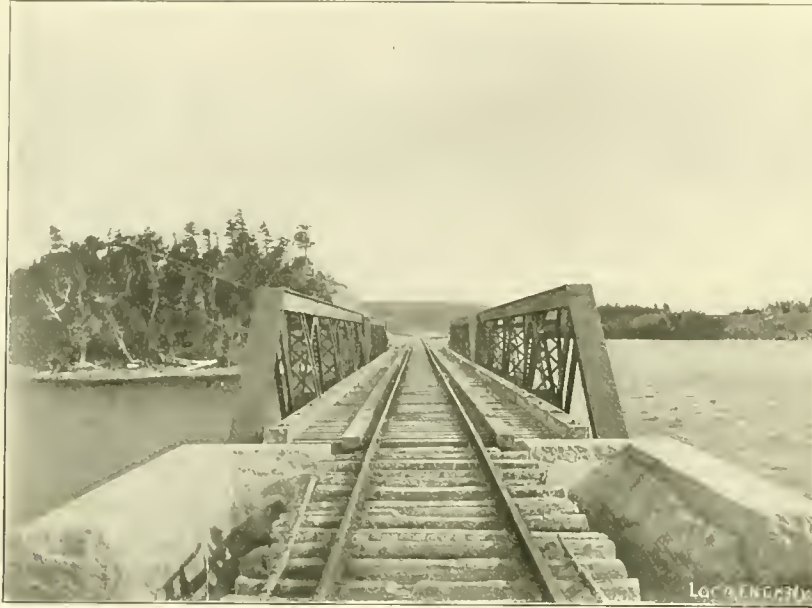
RAILWAY BRIDGE—LITTLE CODROY RIVER.
