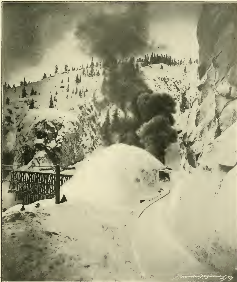
A ROTARY AT WORK ON TUNNEL MOUNTAIN, WHITE PASS & YUKON RAILROAD.
