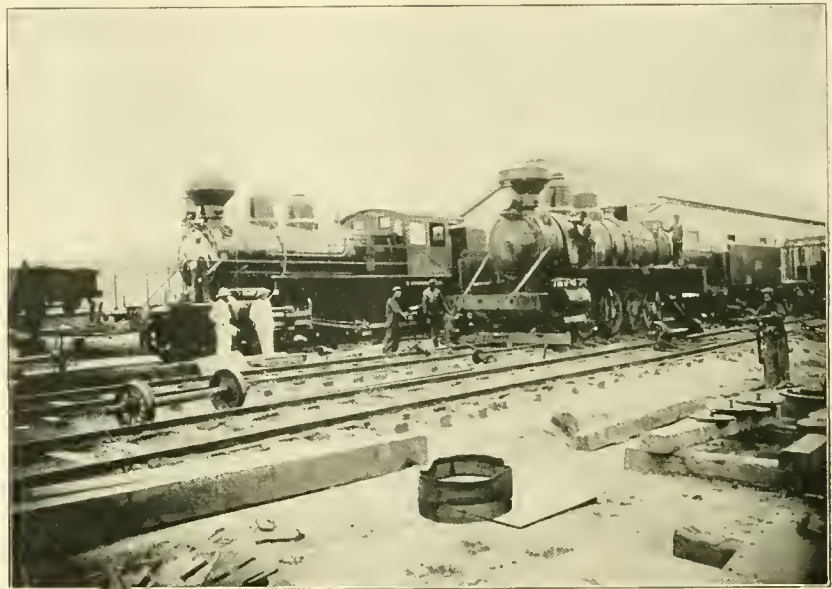
RECTING COMPOUNDS AT VICTORIA BAY FOR CHINESE EASTERN RAILWAY.
