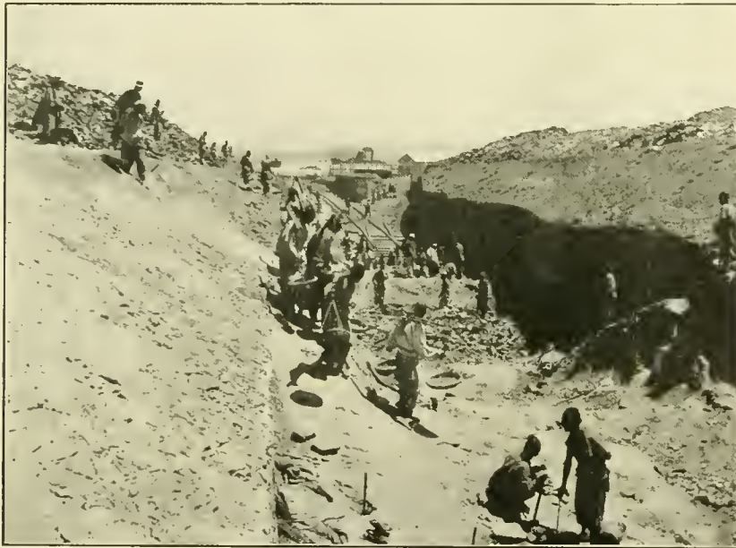
RAILWAY CUT, LOOKING TOWARDS THE BAY.
