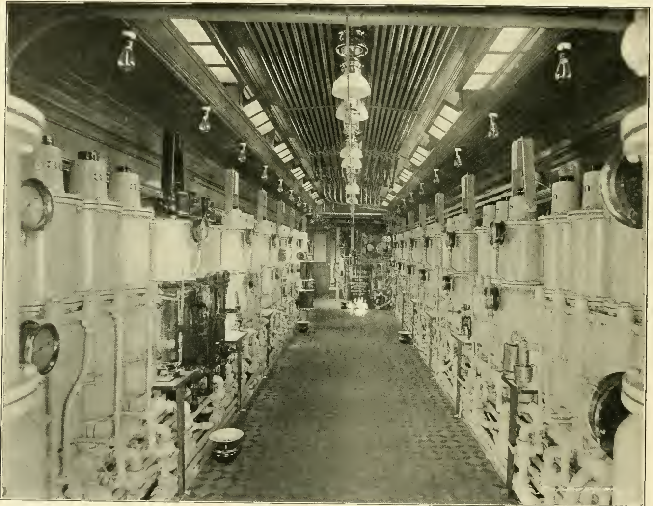
INTERIOR VIEW OF INTERNATIONAL CORRESPONDENCE SCHOOLS' AIR-BRAKE INSTRUCTION CAR, NO. 105.
