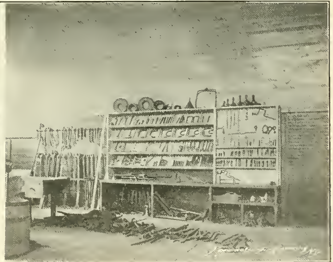
TOOL ROOM IN STORE ROOM.
