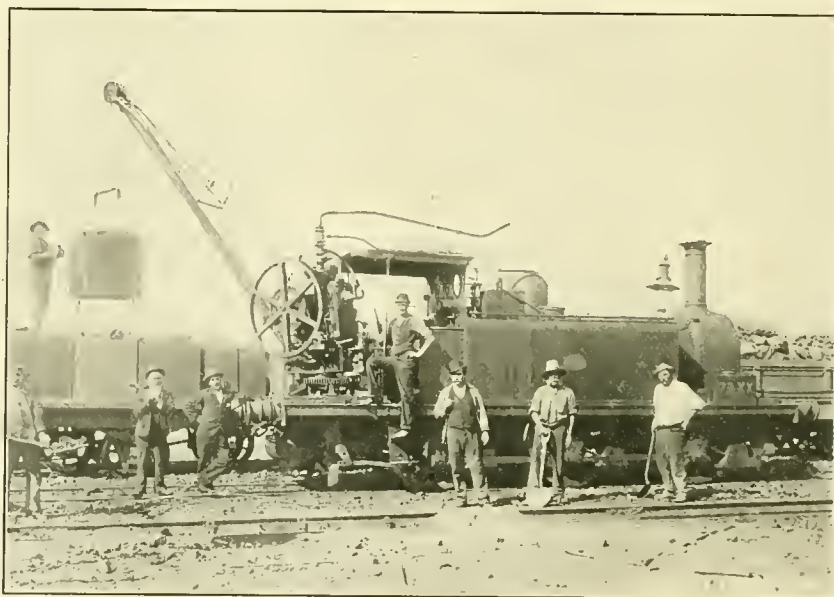
NEW ZEALAND CRANE FOR HANDLING COAL AND CINDERS.
