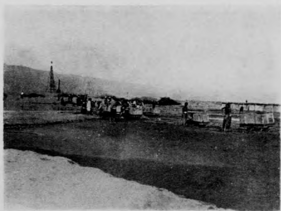
形情作工河引北掘挖
