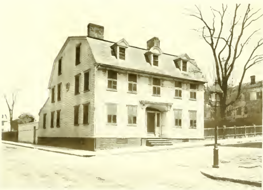
DR. SUTHERLAND'S HOUSE BUILT BY JOHN BASTIER, ESQ., GENERAL OF THE COLY. HEAD-QUARTERS, PELHAM STREET Completed in 1760.
