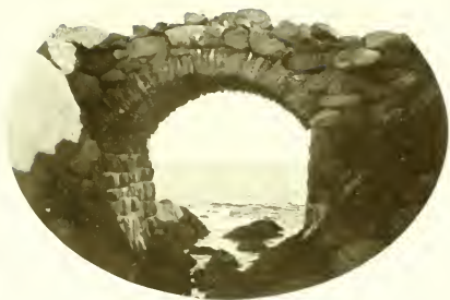
OLD WALK, BRIDGE AT ROUGH POINT
