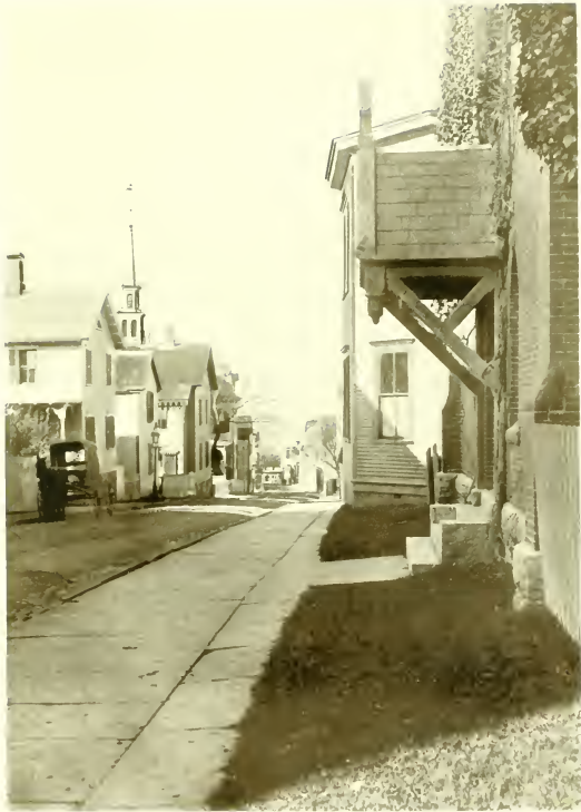
KAY CHAPEL, MASONIC HALL, SPIRE OF TRINITY CHURCH, CHURCH STREET
