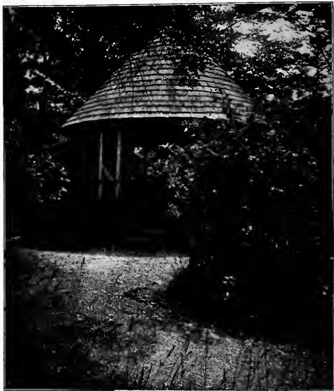
Summer-house at Ravensworth.
