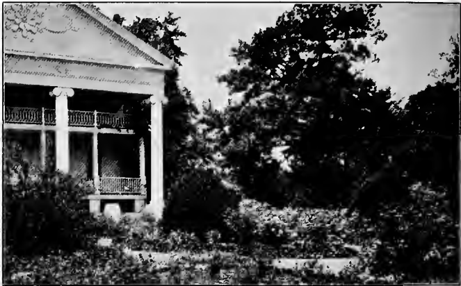
Greenwood, Thomasville, Georgia.
