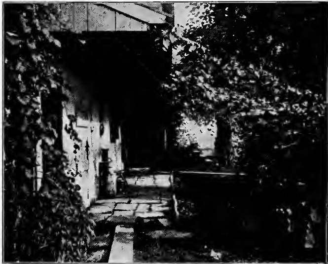
Kitchen Doorway and Porch at the Hedges.
